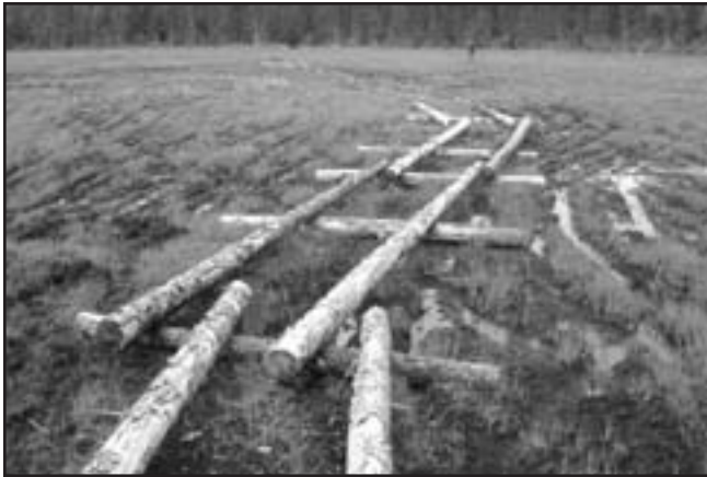
Figure 19—Rough layout of the sill and stringer timbers for puncheon trail construction over a wetland area in southcentral Alaska. Stringers are laid with tops meeting tops and butts meeting butts.
