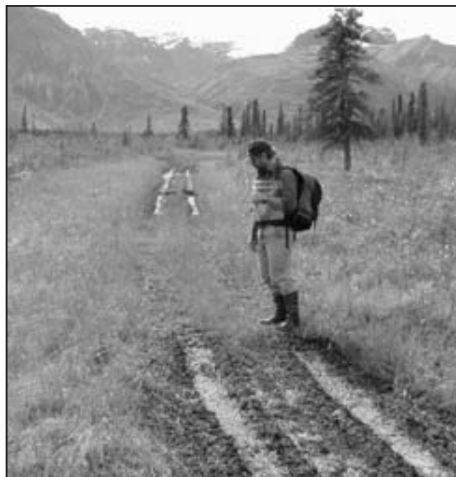
Figure 27—A hardened, protected section of trail 4 years after installation.
