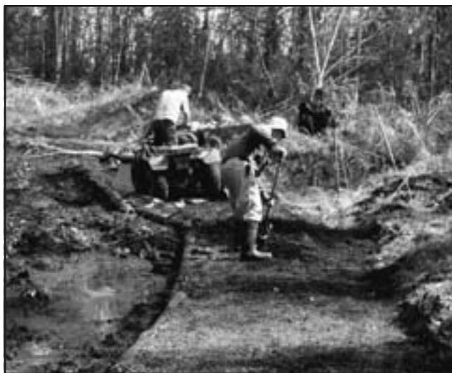
Figure 12—A geotextile and gravel-cap installation over permafrost-degraded soils in Yukon-Charley Rivers National Preserve in Alaska. Use of geotextile and a gravel cap on this trail allowed the National Park Service to construct a 6-foot-wide OHV trail over a 3- to 4-foot-deep muck hole.
