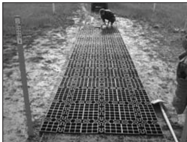
Figure 24—Test installation of SolGrid at the Palmer Hay Flats State Game Refuge in Alaska. Note the U-shaped flex joints between sub-panel sections. The SolGrid was tested without Polynet PN-3000 to test the characteristics of the product when installed on a soft, silty substrate.
