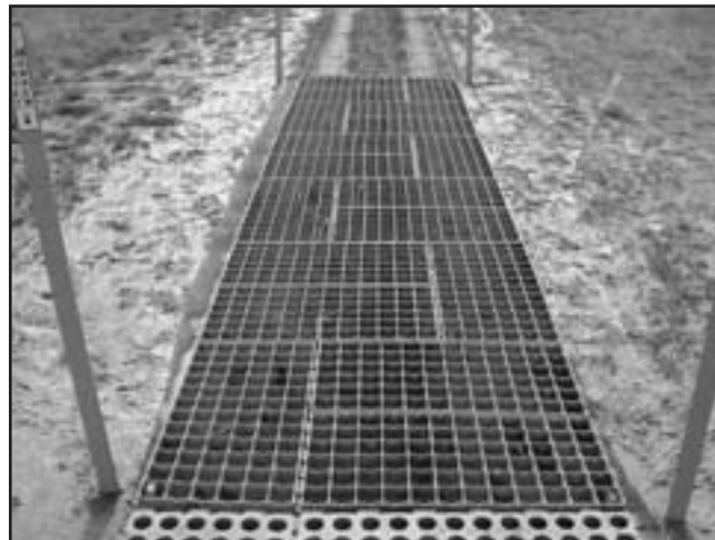
Figure 23—Test installation of 2-inch GeoBlock at the Palmer Hay Flats State Game Refuge in Alaska. This configuration of panels provided a 4.8-foot-wide trail. Note the interlocking tabs along the panel edges. These tabs transfer weight between panels. In this test, GeoBlock was installed over Polynet PN-3000.
