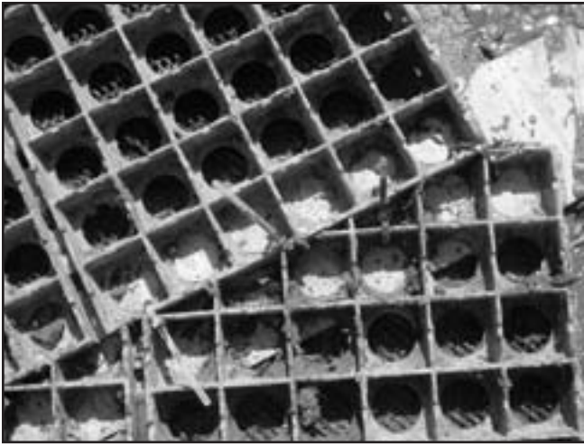
Figure B9—Corner joint showing cut, underlying plywood, and cable ties. Note the screws through the panel's plastic baseplate that secure the panels to the plywood.
