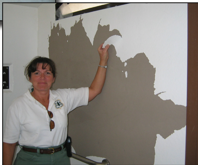
Figure 4—Coatings that come off in sheets are not considered normal. Such problems probably are caused by poor surface preparation or unusual weather conditions.
