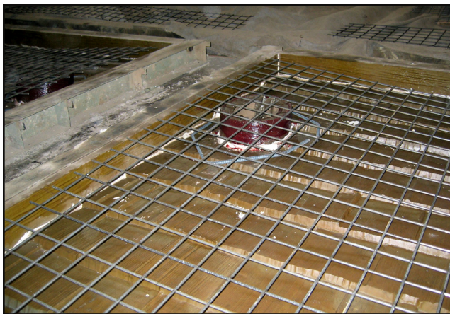
Figure 5—Grids of steel reinforcing bars give strength to concrete panels, lessening the structural concerns that cracks in panels might represent.
