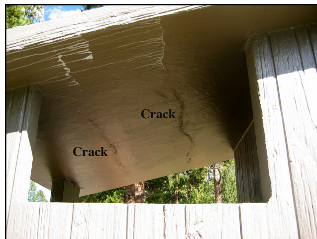
Figure 3—Full-length, full-depth cracks in panels may not be a serious structural concern.
