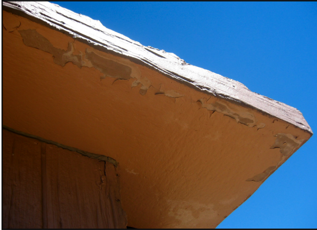
Figure 6—Cracked and peeling paint is common under eaves and around panel connections and joints.
