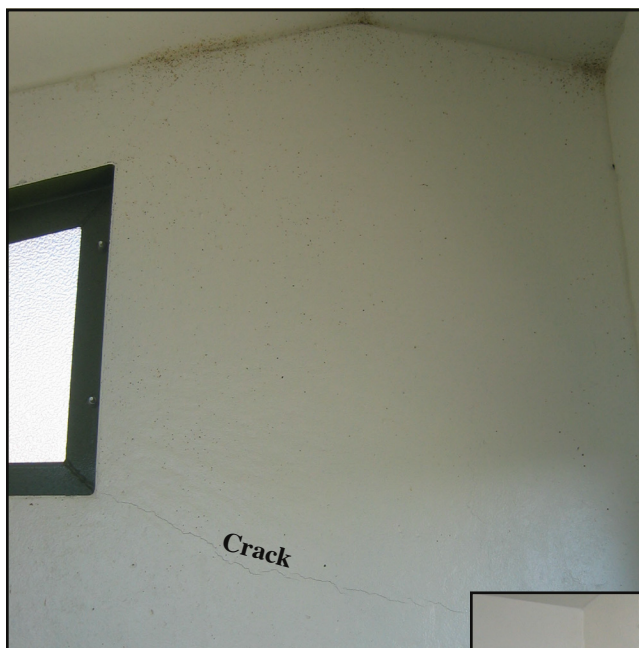
Figure 2—Cracks in concrete typically begin at the sharp edges of doors and windows.
