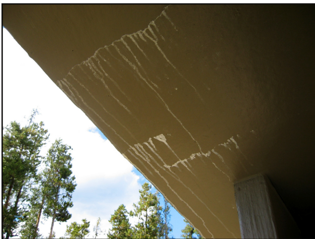
Figure 7—A white, chalky substance called efflorescence found near cracked paint is ugly, but harmless.
