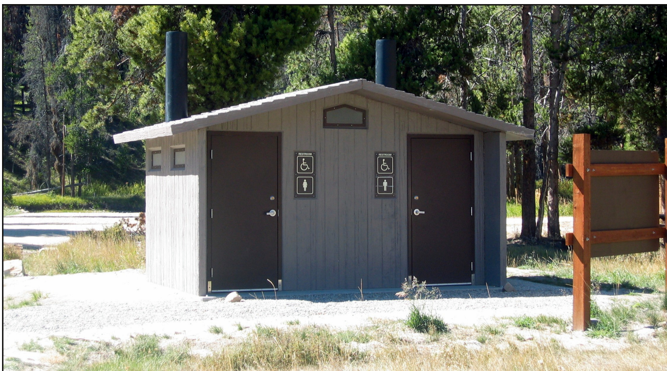
Figure 1—Precast concrete toilets are tough, but still require some periodic maintenance. This Tioga special double-vault toilet is made by CXT, Inc., of Spokane, WA.
