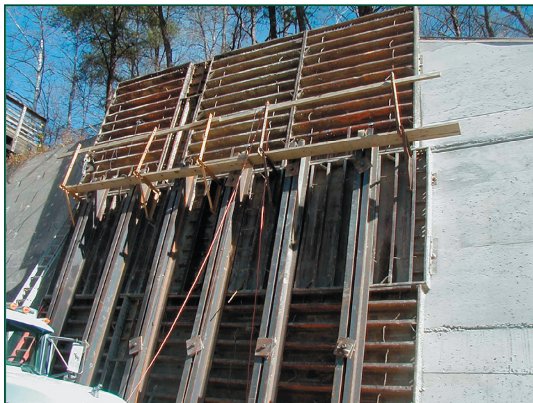
Figure 6—Steel forms used to form spillway walls.
