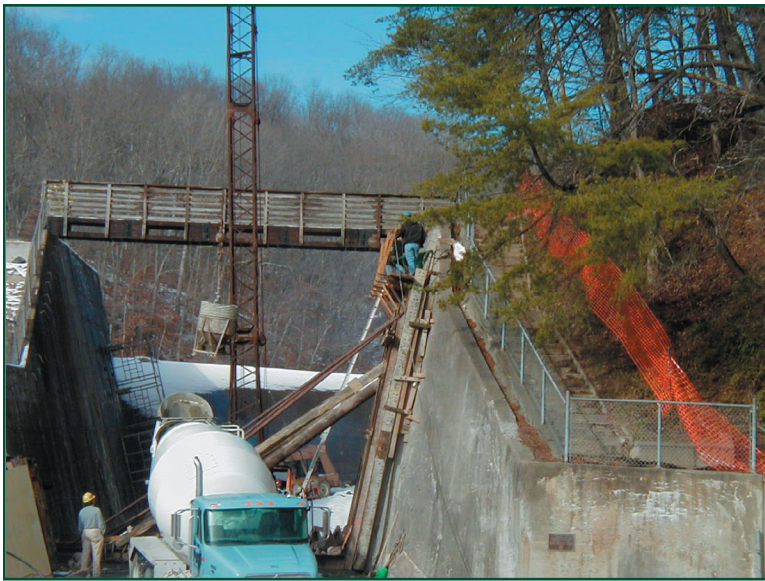
Figure 7—Placement of new concrete overlays of spillway walls using a drop bucket and crane.
