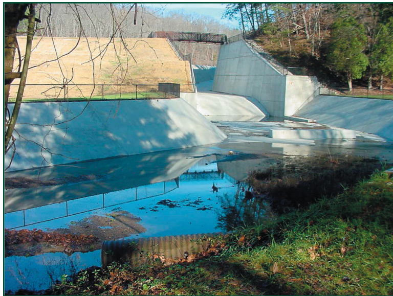
Figure 9—Finished spillway including new stilling basin and partial wier in outlet of spillway.
