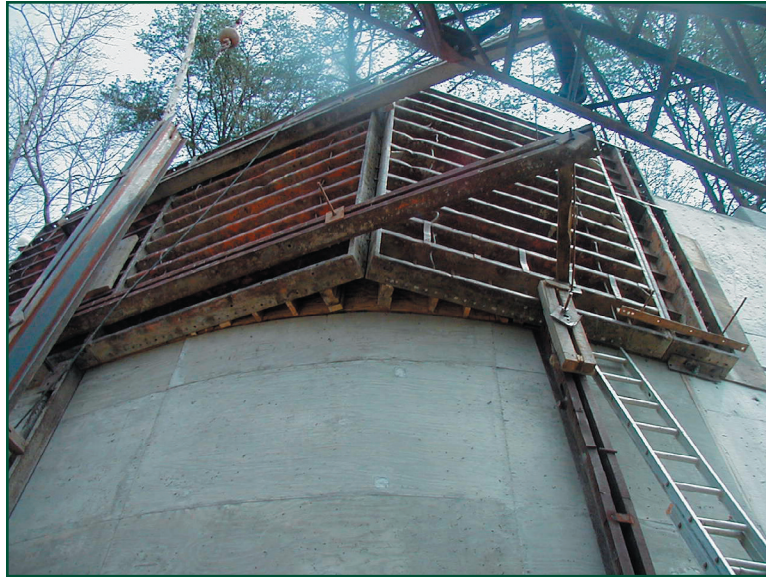
Figure 5—Forming a curved section of spillway wall.
