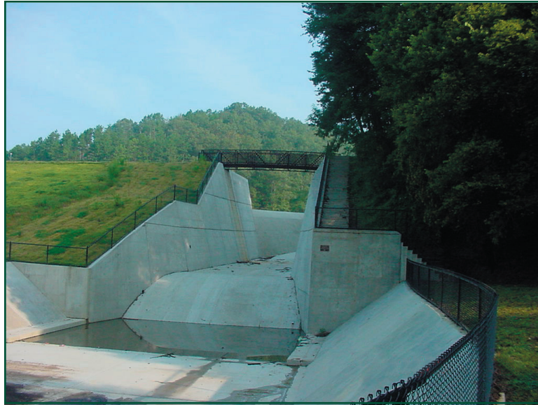
Figure 8—Finished spillway with new trail bridge and fencing installed.
