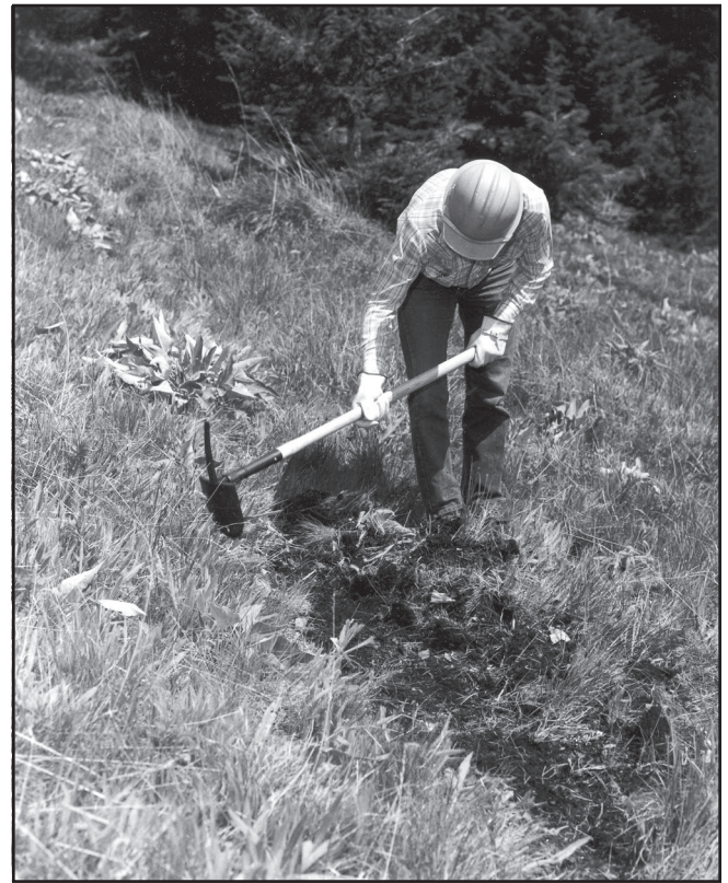
Combination (or Combi) tool developed for firefighting, is popular for trail work.
