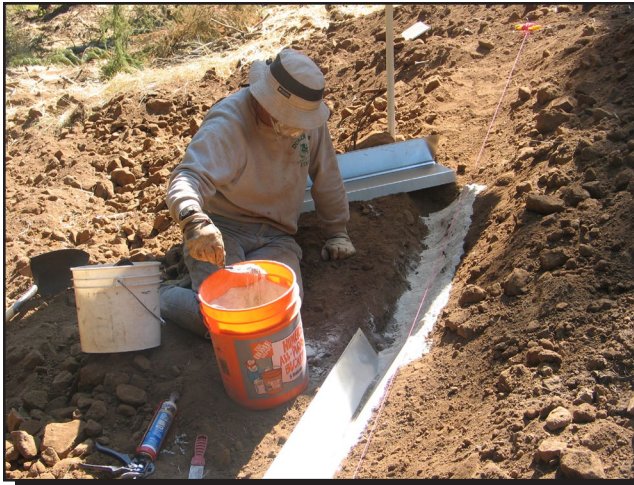
Figure 4—Applying bentonite to seal the trench around the trough.
