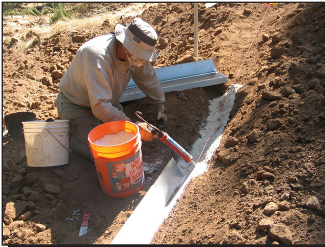
Figure 5—Applying silicone caulking to the trough's overlapping sections.
