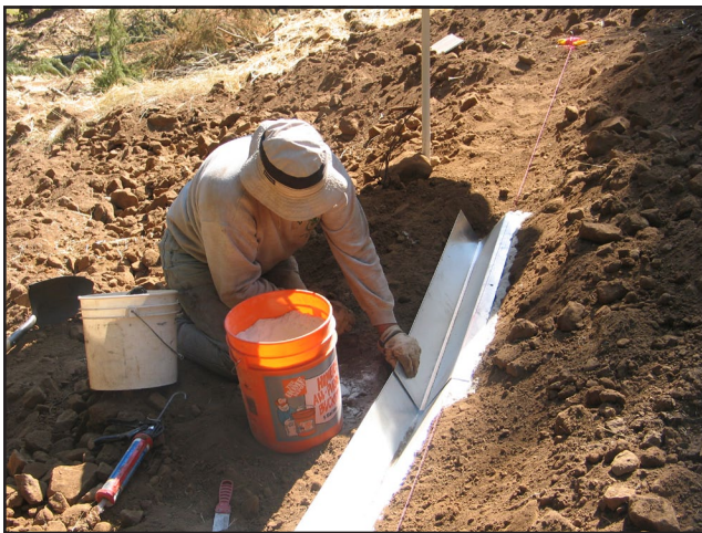
Figure 6—Placing a section of trough in the trench.
