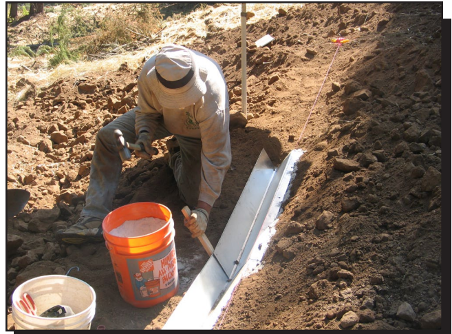
Figure 7—Driving the wooden stakes that hold the sections of trough in place.
