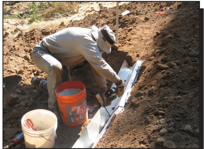
Figure 8—Screwing sections of trough to the wooden stakes.
