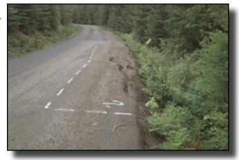
deep patch is a limited-depth earthwork method that uses geosynthetic-reinforced soil materials. The technique is much less expensive than other methods, such as the construction of retaining structures. Deep patching provides a reasonable measure of stability and reduces maintenance costs.
