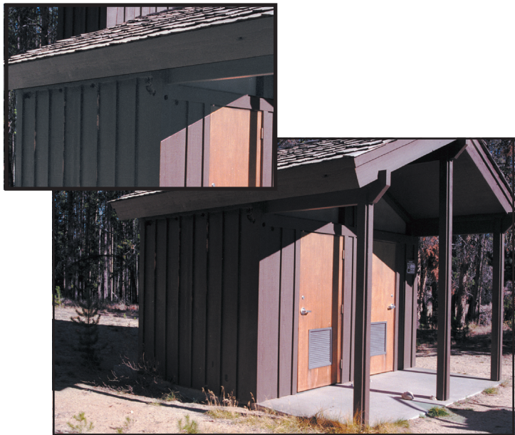
Figure 4—The Pettit Lake vault toilet already had some woodpecker damage when the habanero coating was applied to the left side of the structure in October 2003.
