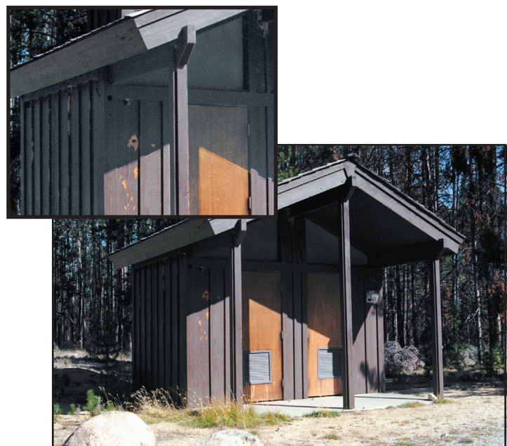
Figure 5—In October 2004, new woodpecker damage was minimal on the left side of the structure, which was treated, but damage was substantial on the front of the building, which was untreated.
