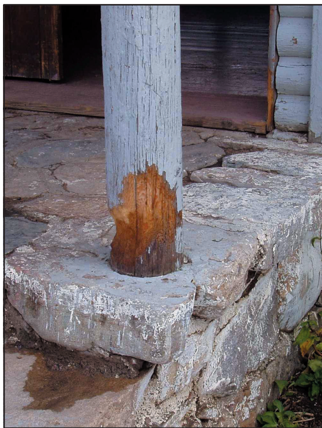
Figure 1 — This porch post at a historic ranger station in the Intermountain Region was damaged by a beaver or porcupine during the winter of 2003–2004.
