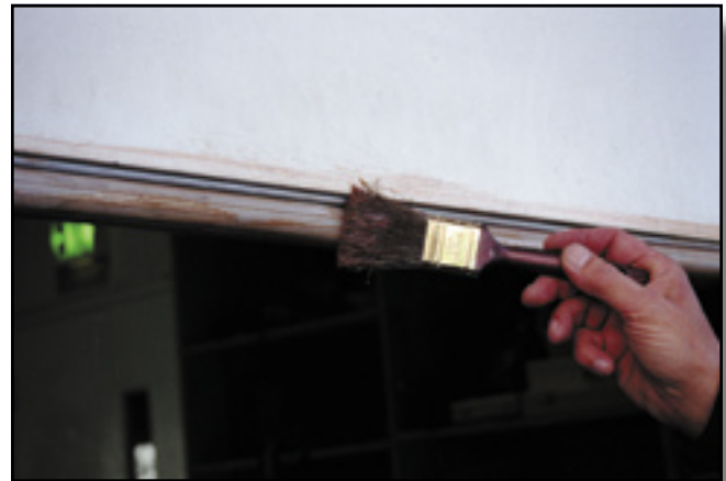
Figure 8—Habanero coating was painted on the overhead door seals at the maintenance shop in the Mount St. Helens National Volcanic Monument. The freshly applied coating had an orange tint, but the coating became clear after several weeks.
