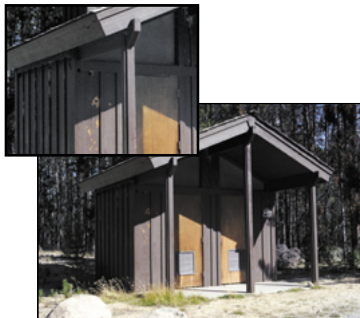
Figure 5—In October 2004, new woodpecker damage was minimal on the left side of the structure, which was treated, but damage was substantial on the front of the building, which was untreated.
