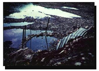
Figure 8-A rounded fence can help keep beavers from damming a culvert.
