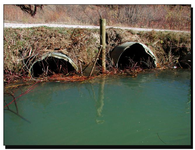
Figure 4-Most culverts create ideal locations for beavers to construct their dams.
