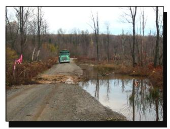
Figure 1—A culvert blocked by a beaver dam on the Allegheny National Forest.
