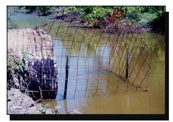
Figure 11—A culvert guard can be constructed by rolling wire mesh panels into cylinders.
