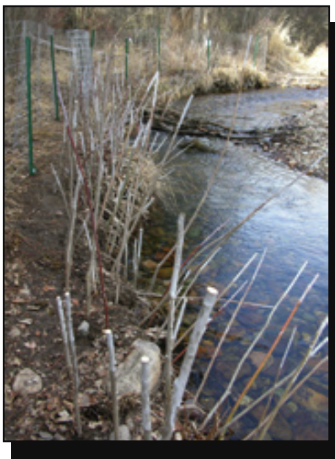
Figure 1—Cuttings were planted to stabilize an eroding creek bank.—Kristi DuBois photo
