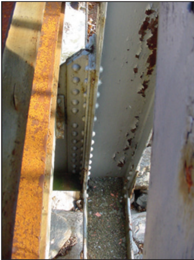
Figure 4—Flaking paint may contain lead or other heavy metals that can present health hazards.
