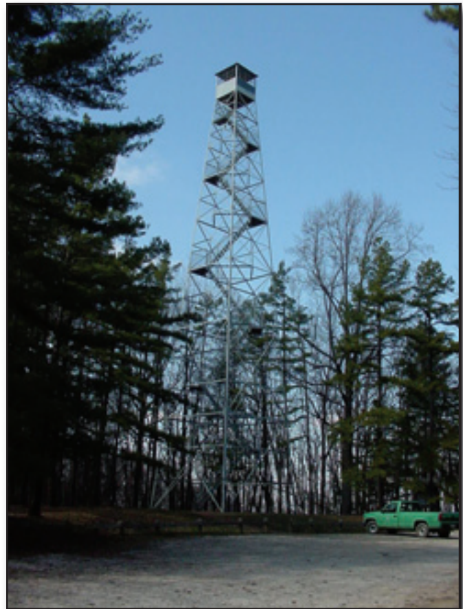
Figure 1—Steel towers may be coated with lead-based paint. Special precautions for climbing won't be needed when taking samples from a tower's lower steps, but samples elsewhere may need to be taken by a certified climber following all appropriate safety guidelines. The same precautions apply to persons taking samples in precarious spots under bridges.
