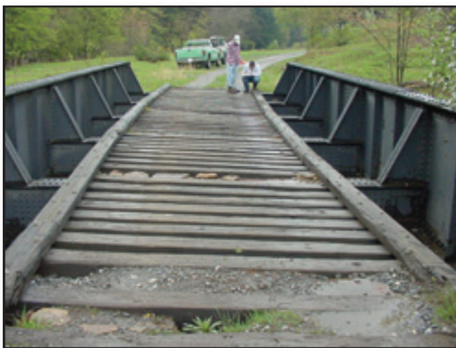
Figure 3—The beginning phase of a project involves onsite inspection to determine whether lead or other heavy metals are present.
