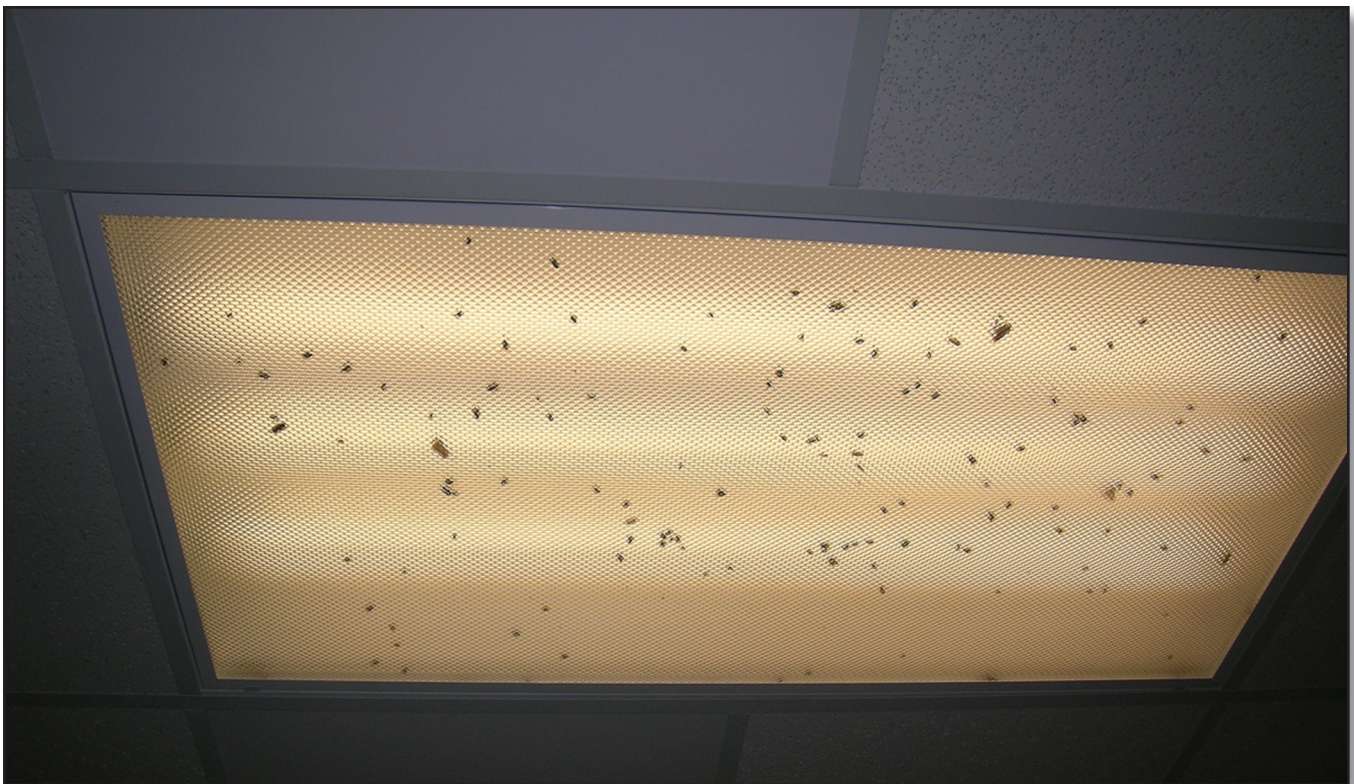
Figure 5—A fluorescent lamp with a luminaire that needs to be cleaned or replaced.
