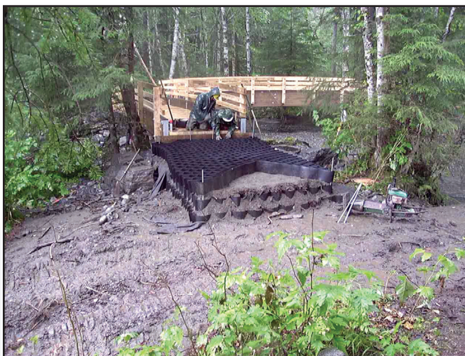
Figure 18—Using geocells to construct a trail bridge approach.
