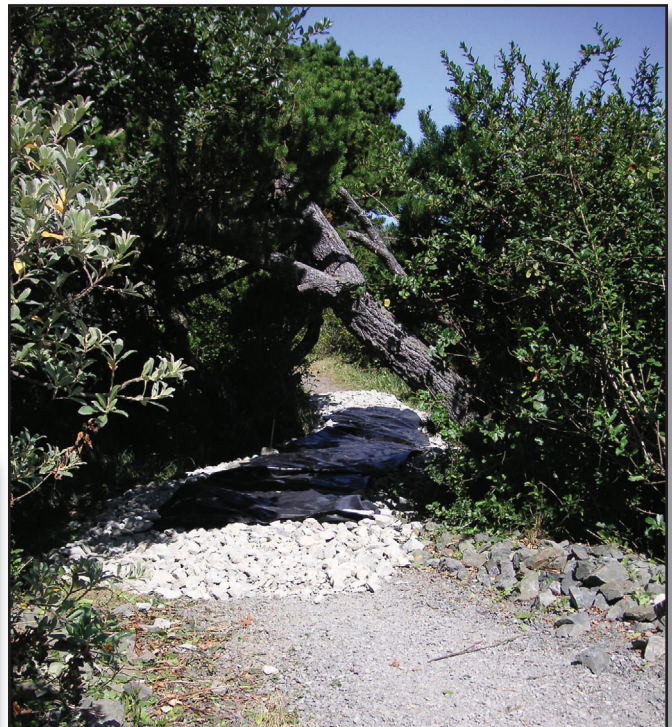
Figure 21—Constructing an underdrain from large rocks, with geotextile serving as a separator between surface material and large rocks.
