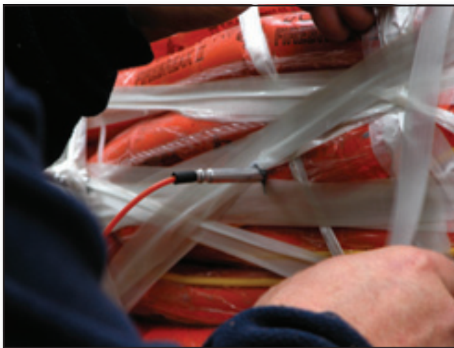
Figure 7—Place a nonelectric blasting cap on top of fireline explosives after they are taped to the outside of a hazard tree.
