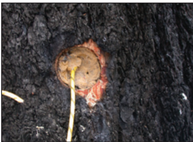
Figure 4b—Noise and airblast can be reduced by loading explosives internally.
