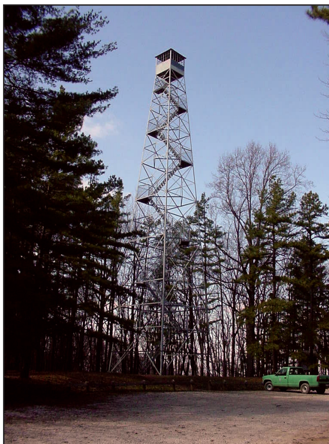
Figure 2—Steel towers may be coated with lead paint buried beneath many other layers of paint.
