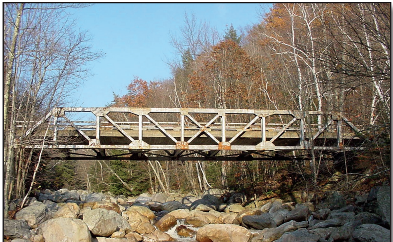
Figure 1—Because steel bridges may be coated with lead-based paint, they need to be tested before restoration or maintenance projects that may disturb the painted surface.
