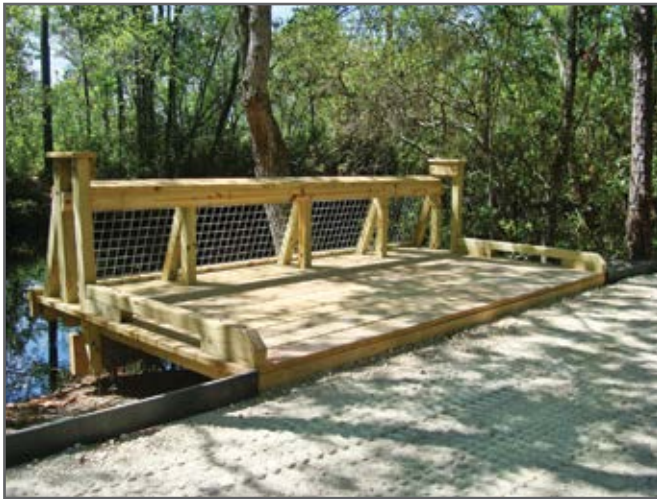
Step 12—Build adjacent trail structures, such as viewing/fishing platforms, so the platform deck height is flush with the adjoining finished trail tread.
