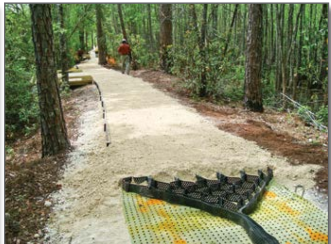
Step 10—Plastic wood borders are not needed for flatter areas.
