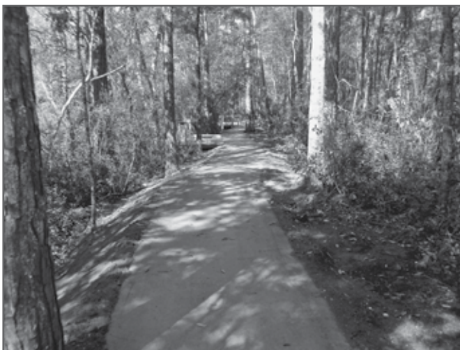
Figure 1—An accessible trail surfaced with NaturalPAVE XL Resin Pavement, immediately after construction.
