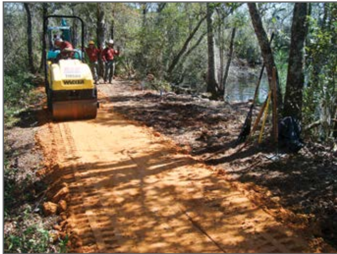
Step 3—Compact all materials with a roller.
