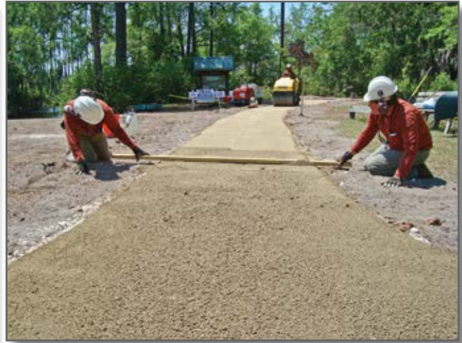
Step 14—Level the surface with a wooden screed, sloping slightly to one side for water runoff.
