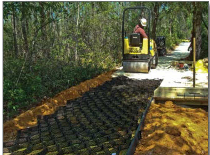
Step 9—Mechanically compact and level the material to the designed depth or cell height.
