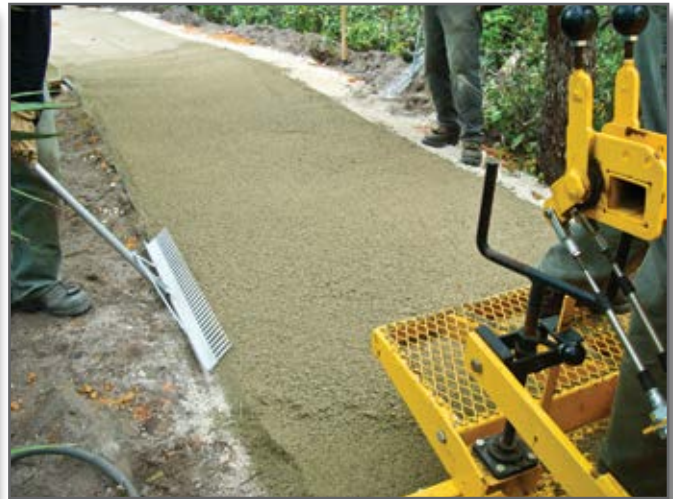
Step 15—Form up the edges with handtools.
