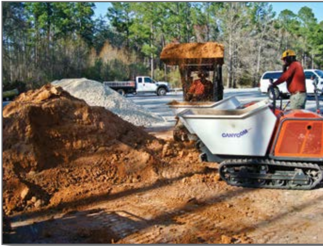
Step 2—Haul in local borrow sand-clay material to spread over poor soils or to increase elevations as desired. Spread, level, and mechanically compact until no signs of displacement are visible.
