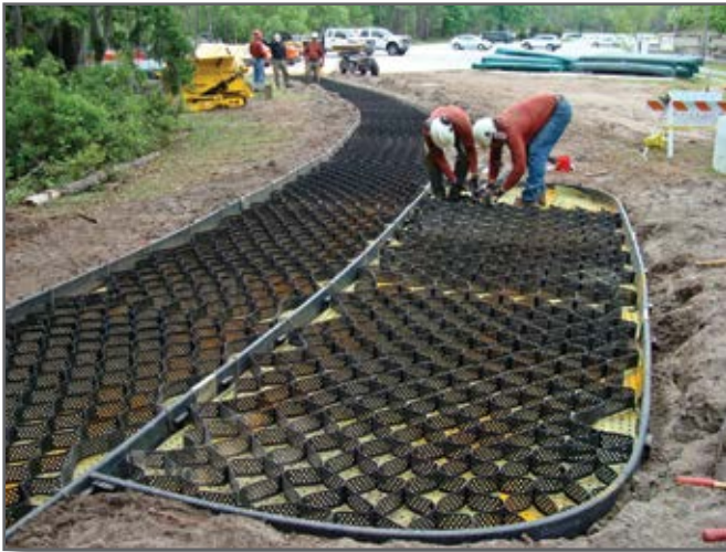
Step 11—Construct any necessary turnouts in a similar manner.
