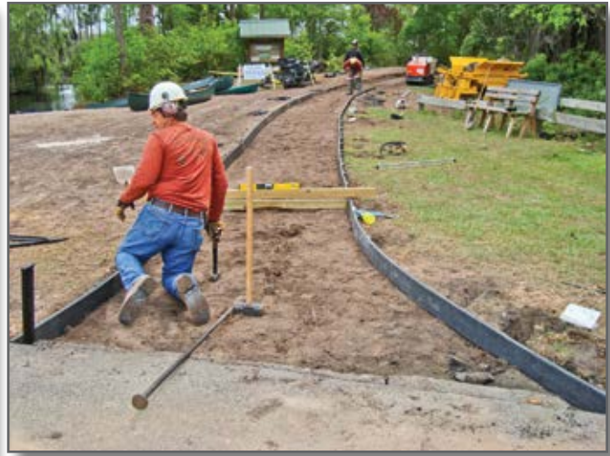
Step 4—Install 5½-inch plastic wood boards on both sides of the elevated portions of a trail where materials and surfacing must be contained in the confined treadway. The boards are secured with three ½- by 24-inch acrylonitrile butadiene styrene (ABS) stakes and will not rot.
