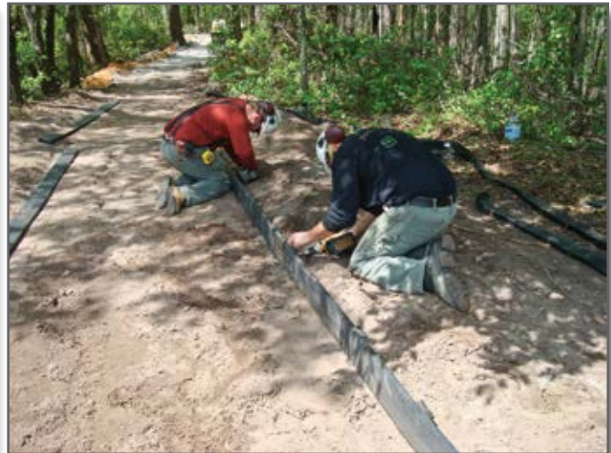
Step 5—Splice the boards together with metal sleeves to minimize movement.
