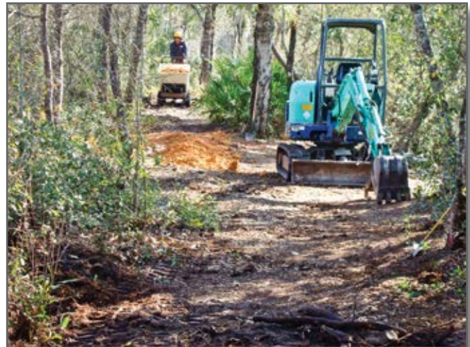
Step 1—Grade the existing ground to the desired width and grade. Remove organic material down to mineral soil.
