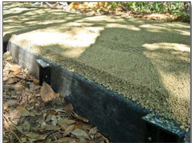
Step 16—Place 2½ inches of NaturalPAVE XL Resin Pavement to acquire a 2-inch thick compacted pavement.
