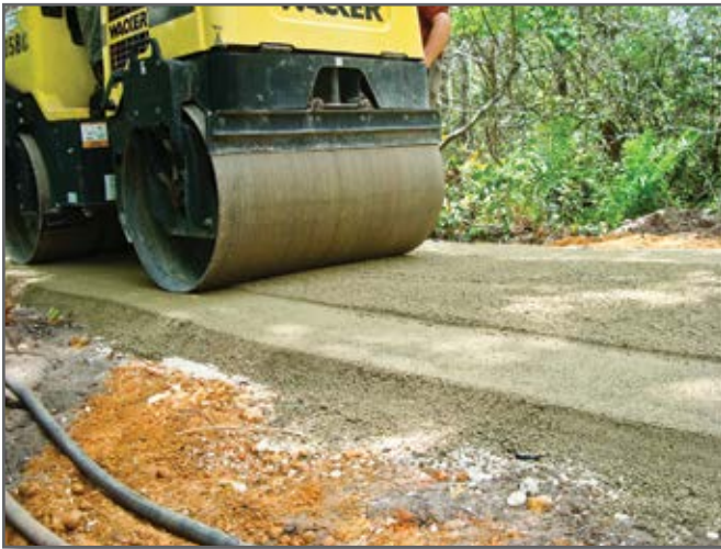
Step 18—Compact the center of the trail with a steel drum roller.
