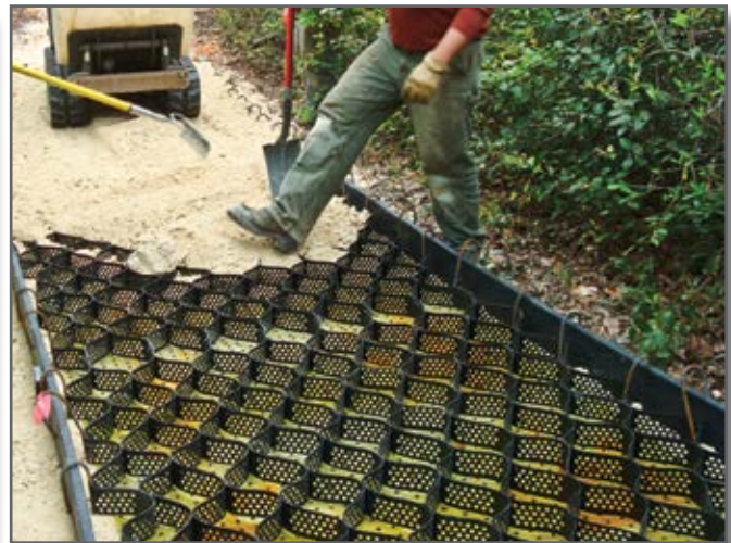
Step 8—Fill the geocells with ¾-inch-minus crushed gravel and spread it evenly throughout the grid.
