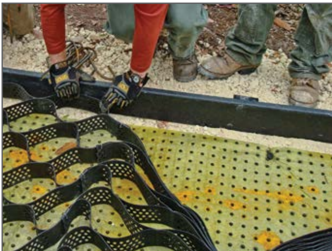
Step 7—Lay 3-inch thick geocell over the Biobarrier or geotextile fabric. The geocell is held to the border with metal clips and keeps the gravel aggregate in place.
