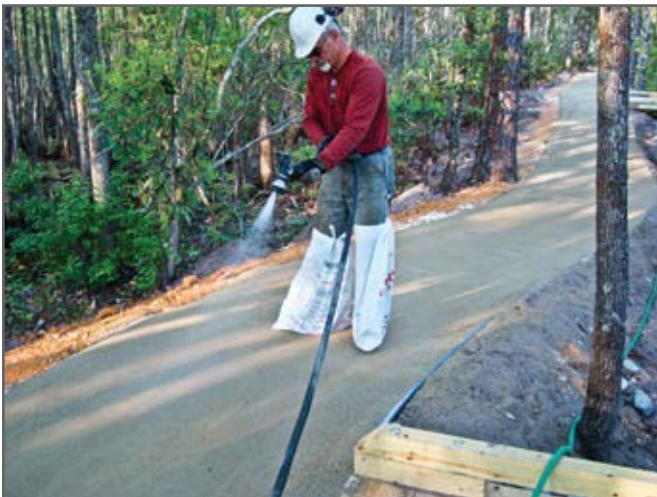
Step 19—NaturalPAVE XL Resin Pavement must be applied during dry weather. Allow the surface to cure for 24 hours, then spray a fog coat sealant over the entire surface using the manufacturer's recommended application rate.
