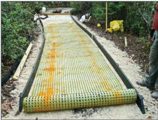
Step 6—Biobarrier geotextile is added next.
