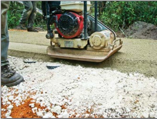
Step 17—Compact the trail edges with a plate compactor. The edges extrude too much if a steel drum roller is used.
