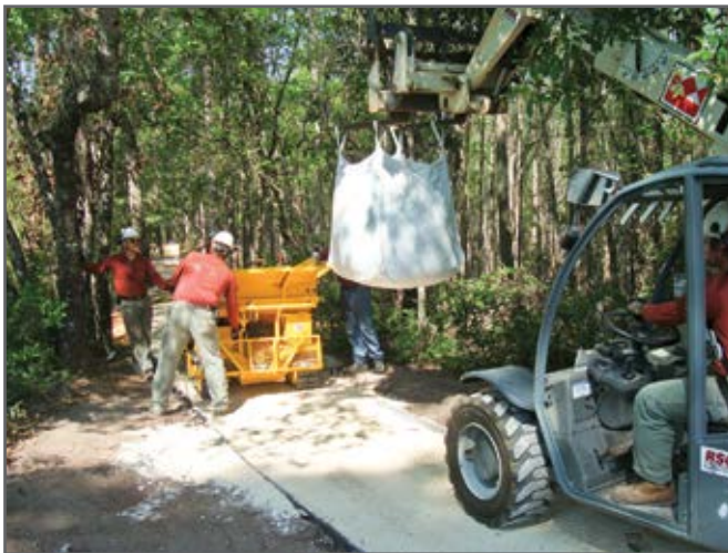
Step 13—Place NaturalPAVE XL Resin Pavement with a small mechanical paver (or by other means) to spread the material.
