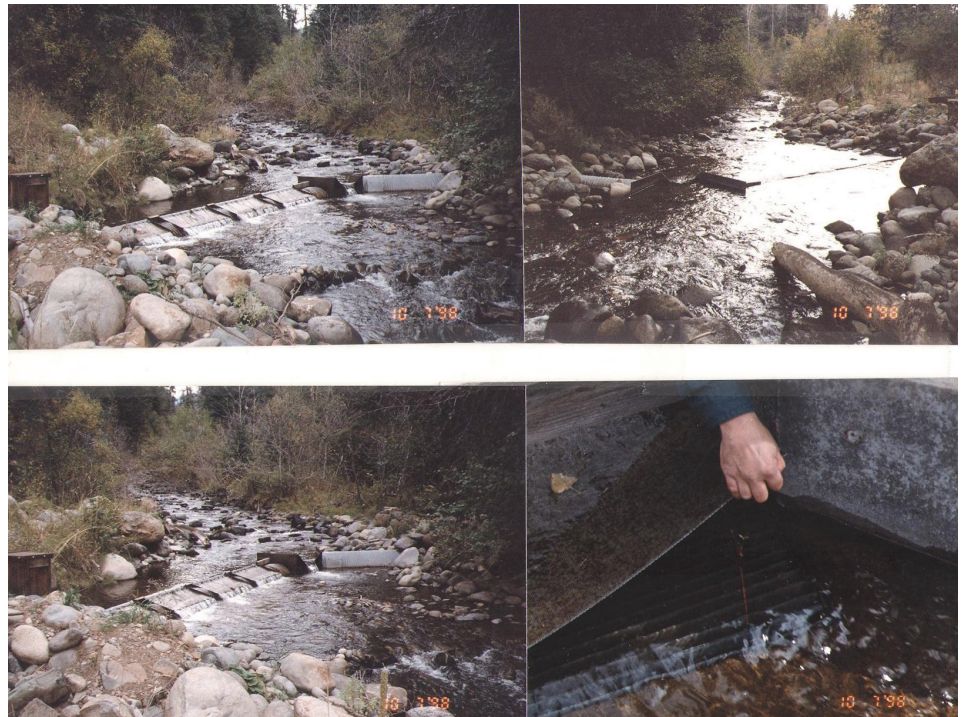
Figure 4.23—Streambed water intake and fish screen on Clear Creek, near Halfway, OR. This structure is a corrugated metal pipe with rectangular holes cut in the top that are covered by a grating. The grating slopes downstream 6 inches in 2 feet (25 percent) so that flow across the top will sweep it clear of debris. This works as long as the grating is submerged, but at low flows, all streamflow may enter at the top and resurface near the bottom, creating a problem for debris and fish passage. Note the piece of culvert at the far side of the stream channel. It acts as a low dam narrowing the channel so that water flows toward the diversion structure. An opening for upstream fish passage can be seen between the two structures.
