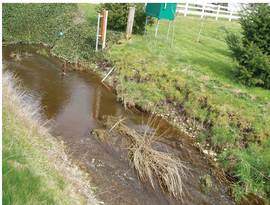
Figure 6.1—Open-channel control section and staff gauge at USGS gauging site on an unnamed tributary of Bertrand Creek, near Lynden, WA (not a diversion ditch). Photo courtesy of Darrin Miller, USGS, Sedro-Wooley WA. This control section is not ideal because of its location downstream of a bend. Preferably, the control reach should be located on a straight section where downstream conditions are relatively unchanging.
