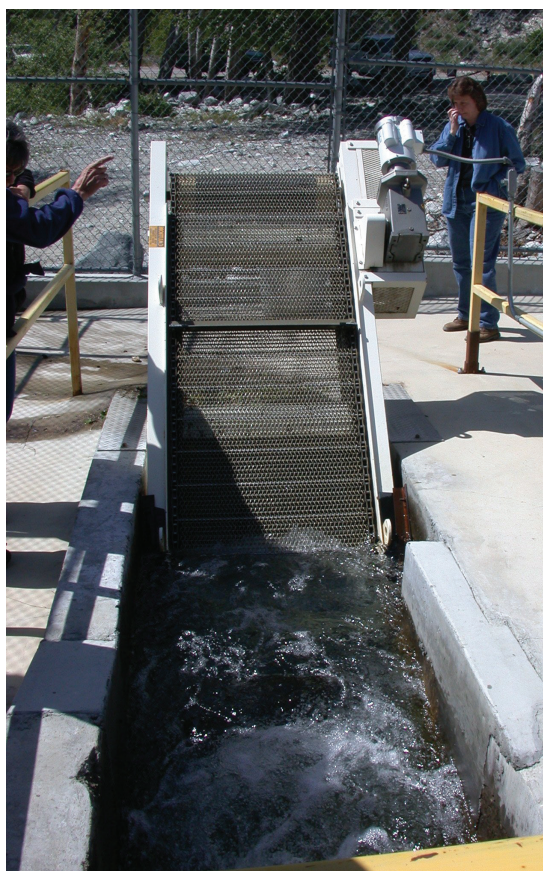
Figure 5.9—Traveling-belt fish screen, Lytle Creek, San Bernardino County, CA, protects a municipal water intake.
