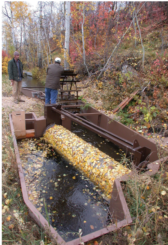
Figure 5.1—Looking downstream at double rotary drum screen installation on Fourth of July Creek diversion, Salmon River Basin, ID.
