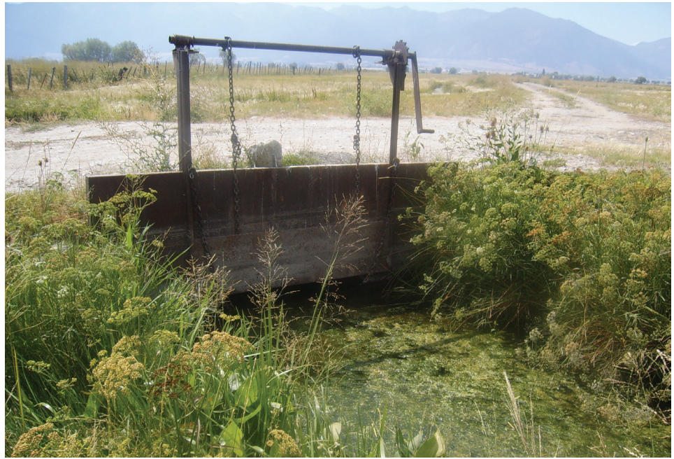
Figure 3.7—Hand-operated windlass headgate, Baker Valley, OR.
