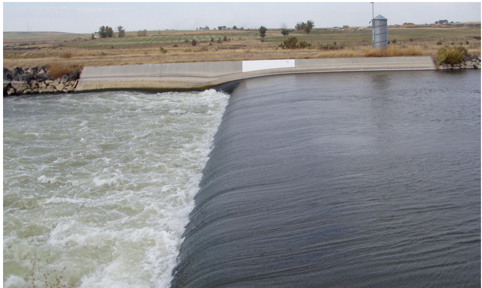
Figure B.2—Broad-crested weir on the Twin Falls main canal, Murtaugh, ID. This is the main measuring device for the Twin Falls Irrigation District. It is remotely monitored by telemetry and is powered by solar panels. Telemetered data from this site is used to adjust upstream head gates to regulate flow to a setpoint that is monitored at this weir. A setpoint is simply the target gauge reading or flow that is required.
