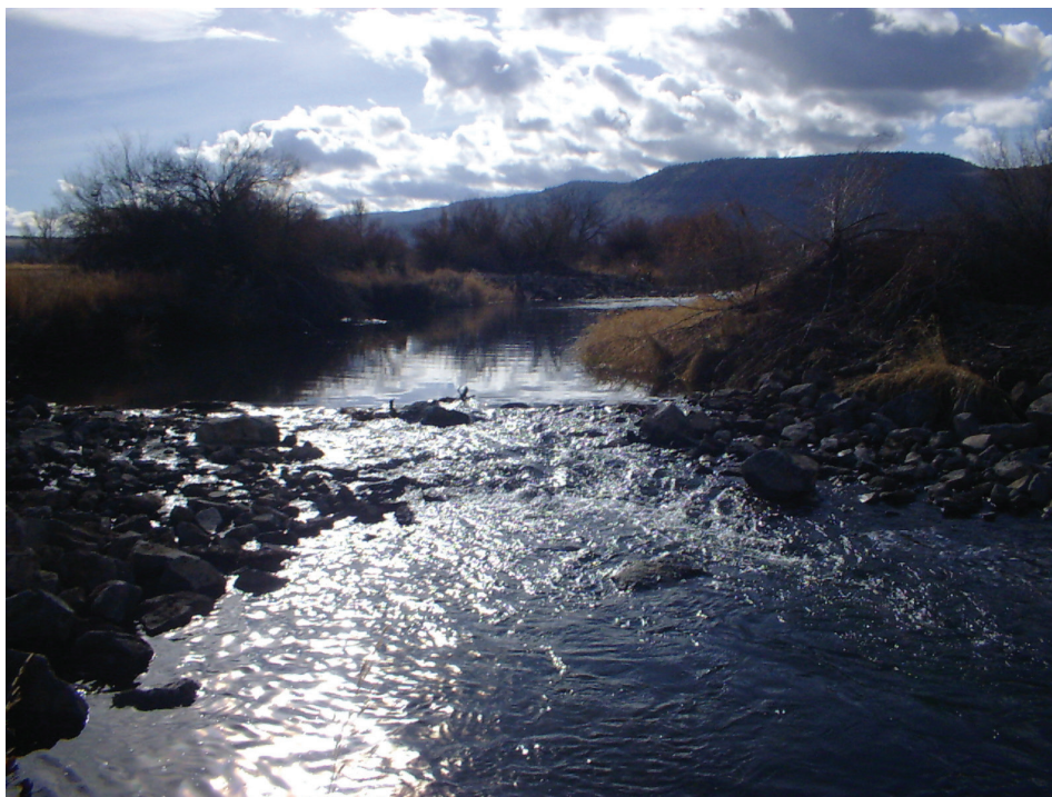
Figure 4.6—Rock weir diversion structure on Donner and Blitzen Creek, OR. Note the low-flow notch in the center that concentrates flows and allows fish passage.
