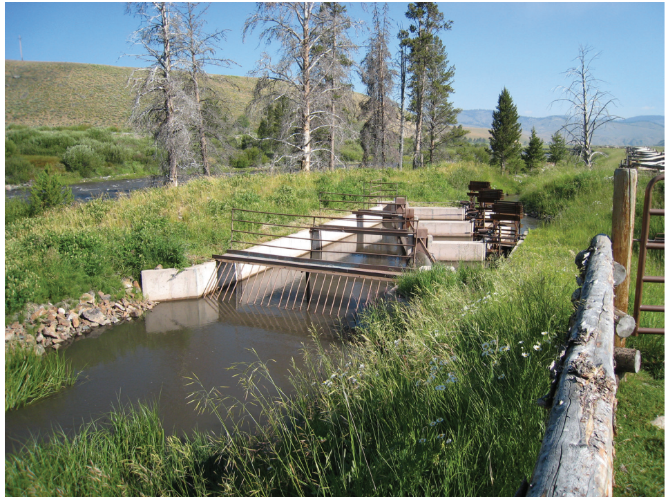
Figure 5.7—Three-bay rotary-drum screen on Salmon River, ID, 2008. Each water wheel powers one drum screen. These permanent concrete installations were common in Idaho until the less expensive, prefabricated versions were developed.
