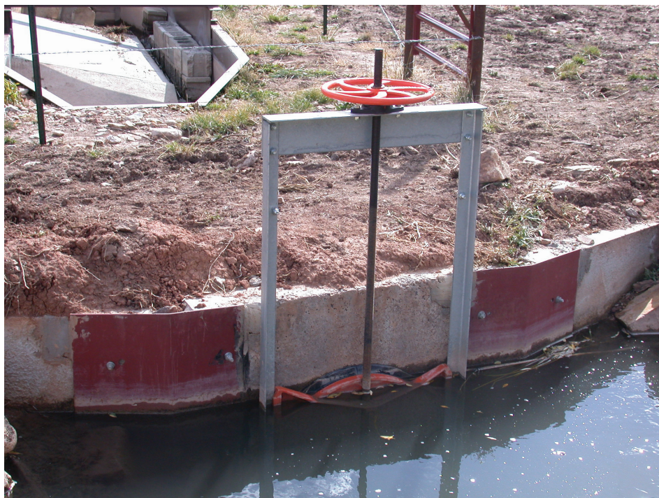
Figure 3.6—Headgate mounted on pipe with concrete headwall and wingwalls, Rock Creek, Bear Lake watershed, WY. A fish screen is in the background.
