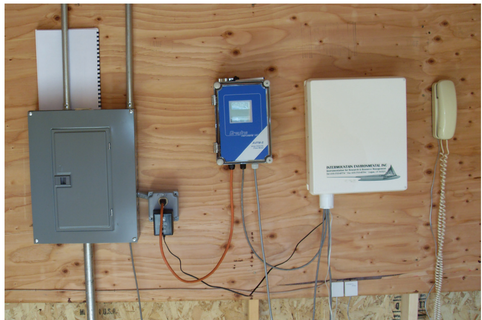
Figure B.4—SCADA components for Middle Cub River diversion, ID. From left to right: the breaker panel for alternating current grid power, the flow meter local readout (blue), and the RTU. The RTU reads the flow from the flowmeter and adjusts the automated gate to maintain the flow at the programmed setpoint. Note the telephone: The irrigation district can call in to the RTU and check the flows, gate position, and make adjustments to the flow setpoint without visiting the site.
