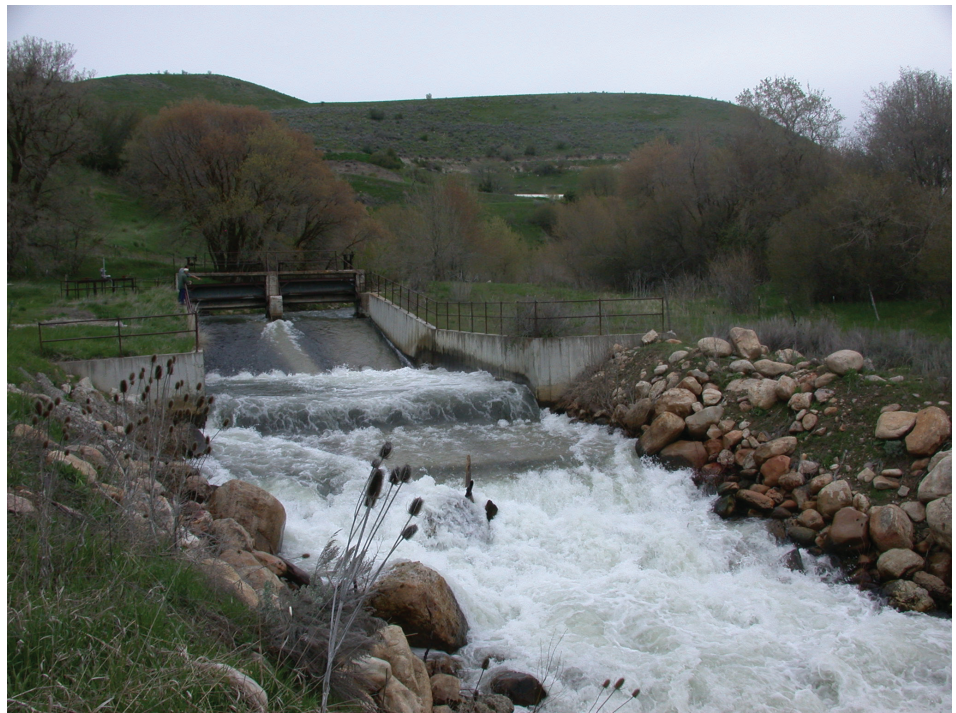
Figure 4.3—Very high velocity water running down this concrete apron caused substantial local scour where the apron met the stream, and another flatter apron was added. Now, the channel has downcut below the second apron. This site is also affected by system-wide channel incision, which has been stopped by the diversion structure. Lower Cub River diversion, Bear Lake watershed, ID.
