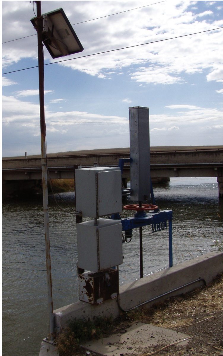
Figure B.3—Automatic gate at Twin Falls main canal, Murtaugh, ID. From left to right---solar panel and antenna; three boxes containing the RTU; regular screw type gate with the actuator, and a cover over the gate stem. The tube running along the back of the concrete head wall goes to a water surface level sensor that measures how much water is flowing through the gate.
