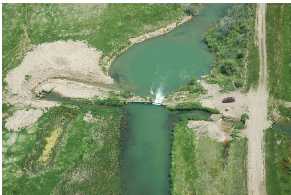
Figure 5.11—Newly constructed open-channel fishway around diversion dam on Thomas Fork, a tributary of Bear Lake, ID. The dam in this photo is 6 feet high, and it backs water up 4 miles. Fishway grade is 3 percent. Stoplogs control flow in the fishway. During the first 2 years of monitoring, this new channel passed not only target salmonid species, but also several native fish species generally considered to be less adept swimmers, including sculpins, suckers, chubs, and over 15,000 speckled dace and redbside shiners (Colyer 2010).
