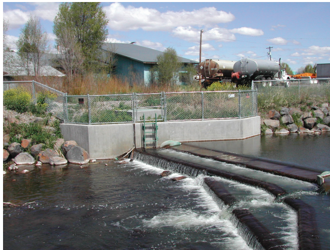
Figure 4.12—Steel weir, Ochoco Creek, Crook County, OR. Note the low-flow notches in the center designed to concentrate flows and allow fish passage. The structure has multiple low steps to facilitate juvenile fish passage and dissipate energy.
