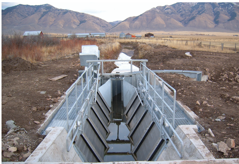
Figure 5.5—Inclined-plate fish screen cleaned by wipers powered by a paddlewheel, Thomas Fork, Bear Lake County, ID. Flow is away from the photographer. This screen serves a 40 cfs diversion. Design and construction cost $150,000 in 2008.
