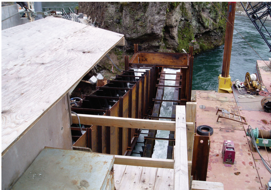
Figure 5.12—Denil steppass fish ladder. This ladder functioned during reconstruction work at the Rivermill dam on the Clackamas River, OR.
