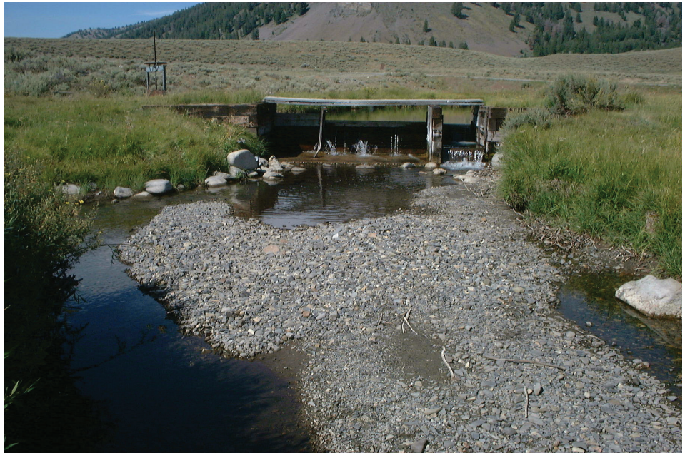
Figure 4.2—Adjustable stoplog weir, Pole Creek diversion, Sawtooth National Recreation Area, ID. Flashboards control water surface elevation behind dam and waterflow to the diversion (left behind wingwall) and fish ladder (right). The structure has a concrete pad upstream and brace downstream to avoid sliding or overturning.
