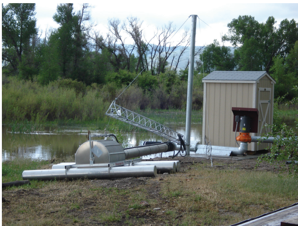
Figure 4.25—Streambank pump with floating screened pump suction on Bear River, UT. Photo courtesy of Warren Colyer, Trout Unlimited.
