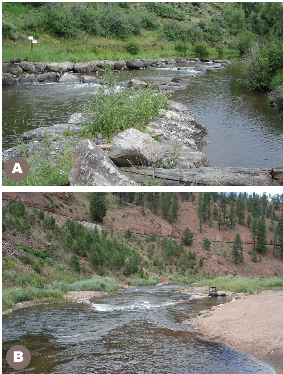
Figure 4.7—(A) Constructed rock steps raise the water surface to headgate elevation at Three Forks Ranch on the Little Snake River, ID. (B) Cross-vane diversion structure, Wigwam Fishing Club, South Fork Platte River, CO.
