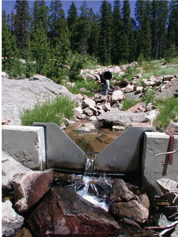
Figure 6.2—Triangular sharp-crested weir on Medicine Bow National Forest measuring instream flow after water is diverted to municipal water intake.
