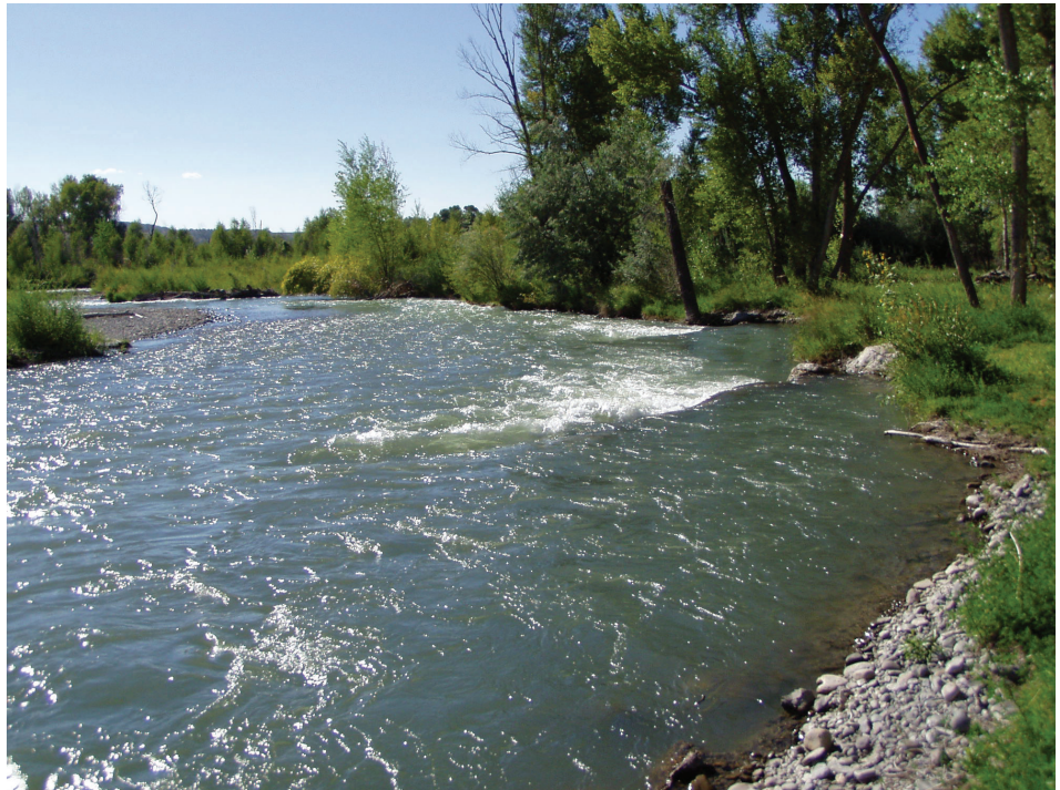
Figure 4.9—Rock barbs bracket a diversion channel on the Uncompahgre River, south of Montrose, UT. The barbs were placed to protect the headgate (not pictured).
