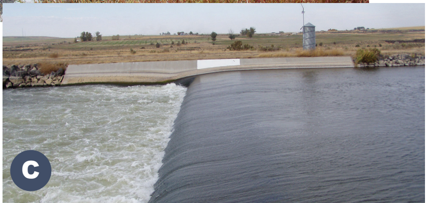
Figure 6.4—Long-throated flume. (A) drawing. (B) Salmon Falls Canal, west of Rogerson, ID. (C) Twin Falls main canal below Milner Dam, ID.
