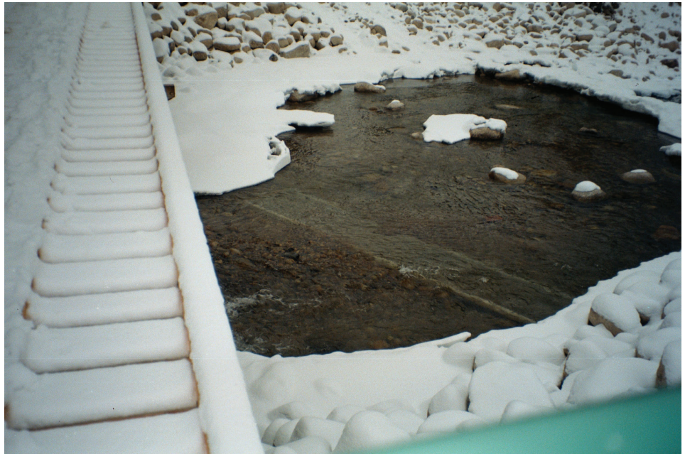
Figure 4.22—Streambed grated intake structure in Boundary Wildlife Management Area, Boundary Creek, ID, operating at low winter flow. This structure is operated by hand to maintain instream flows; no water is diverted at flows less than 50 cubic feet per second (cfs). Permissible diversion rates vary depending on flow in the main channel, and the maximum permissible rate is 20 cfs.
