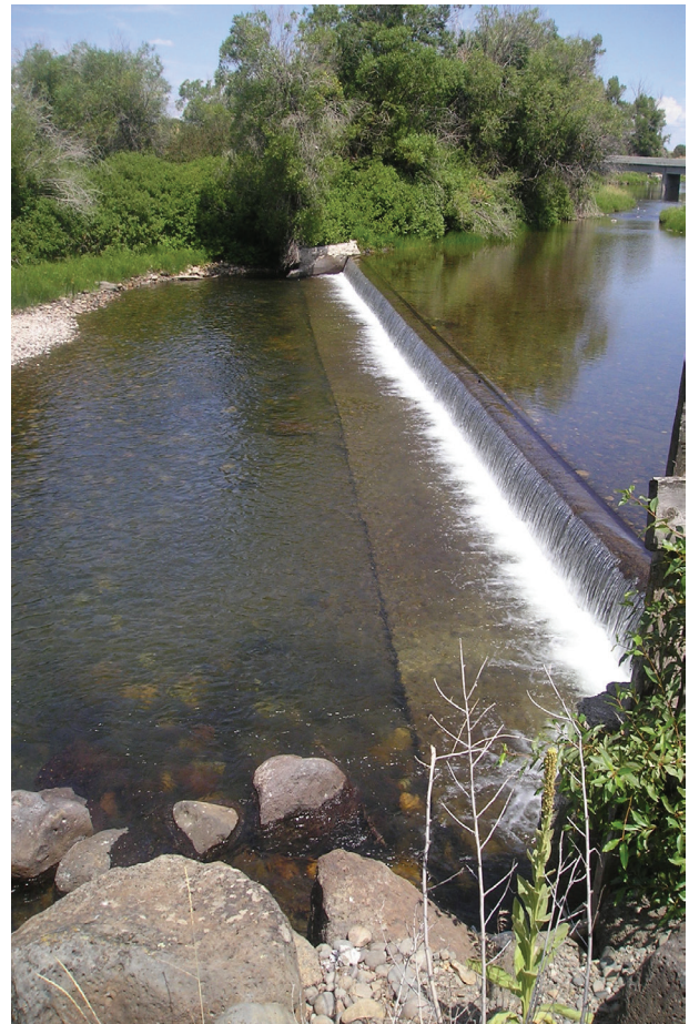
Figure 4.1—Permanent concrete weir drop structure on Fall River, tributary of Henry's Fork Snake River, ID. Photo courtesy of Henry's Fork Foundation, Ashton, ID.
