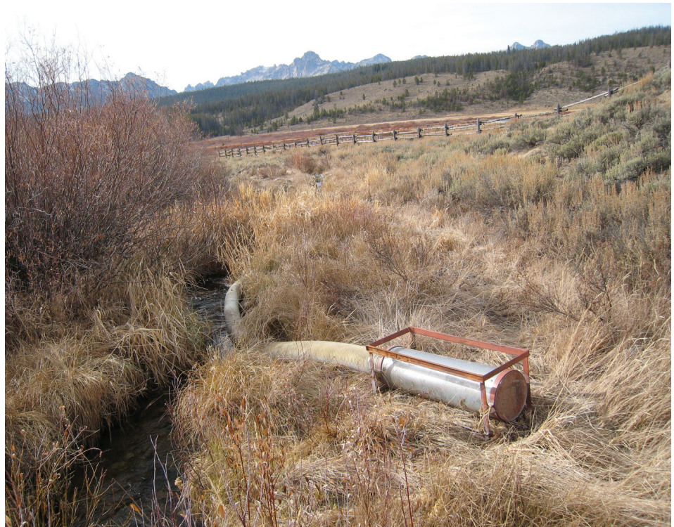
Figure 5.10—End-of-pipe fish screen, Williams Creek, Sawtooth National Recreation Area, ID. This appears to serve a gravity diversion rather than a pump.
