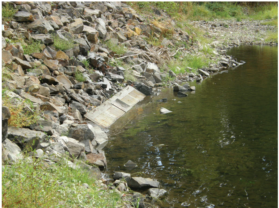
Figure 4.24—Bank screen protecting pump station located behind bank, Kalapuya (also spelled Calapooia) River, near Brownsville, OR.
