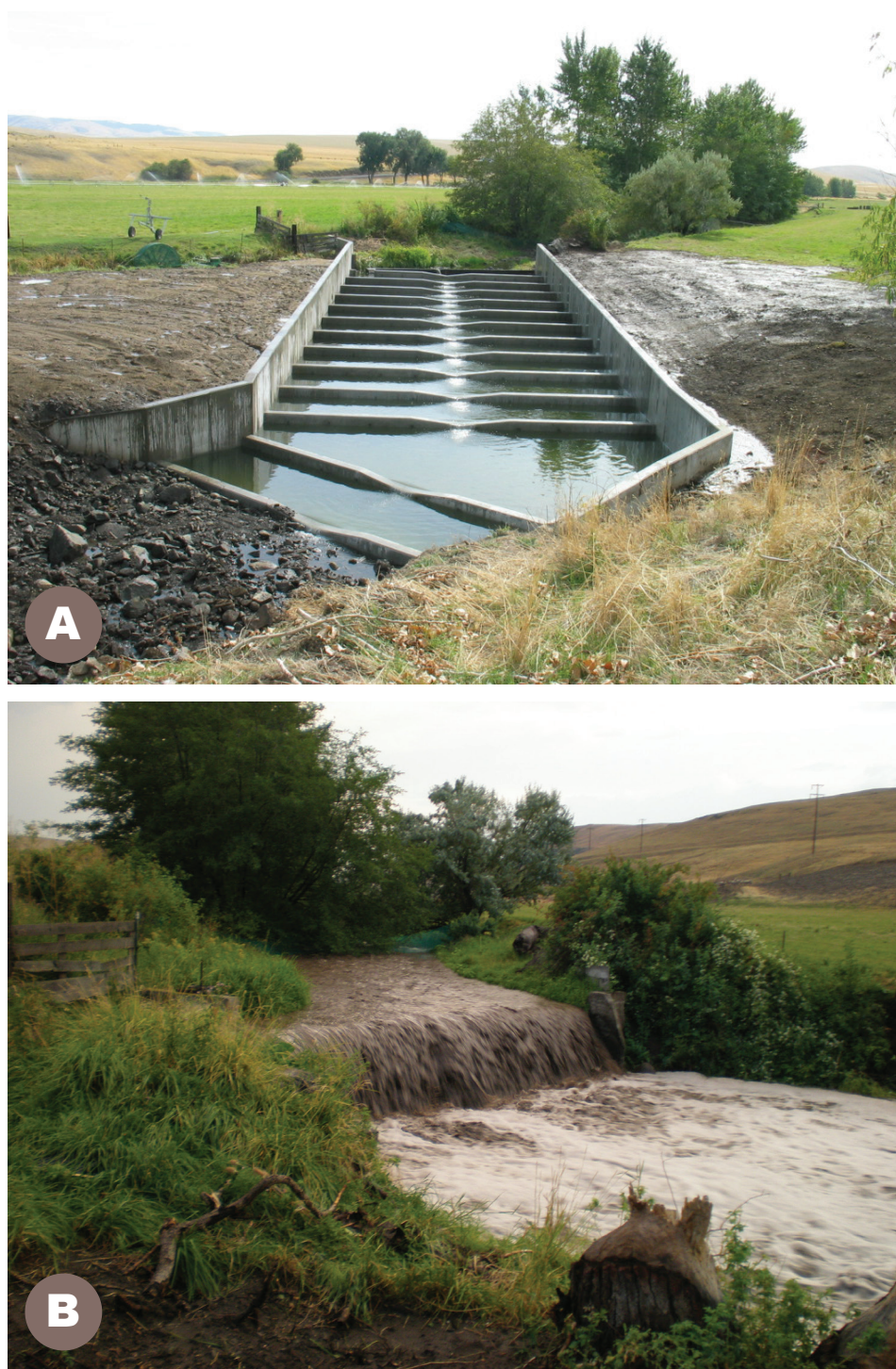
Figure 4.30—(A) Fish-passable pool and weir diversion structure constructed in 2008 on East Fork Birch Creek, OR. (B) The old check structure at the same site.
