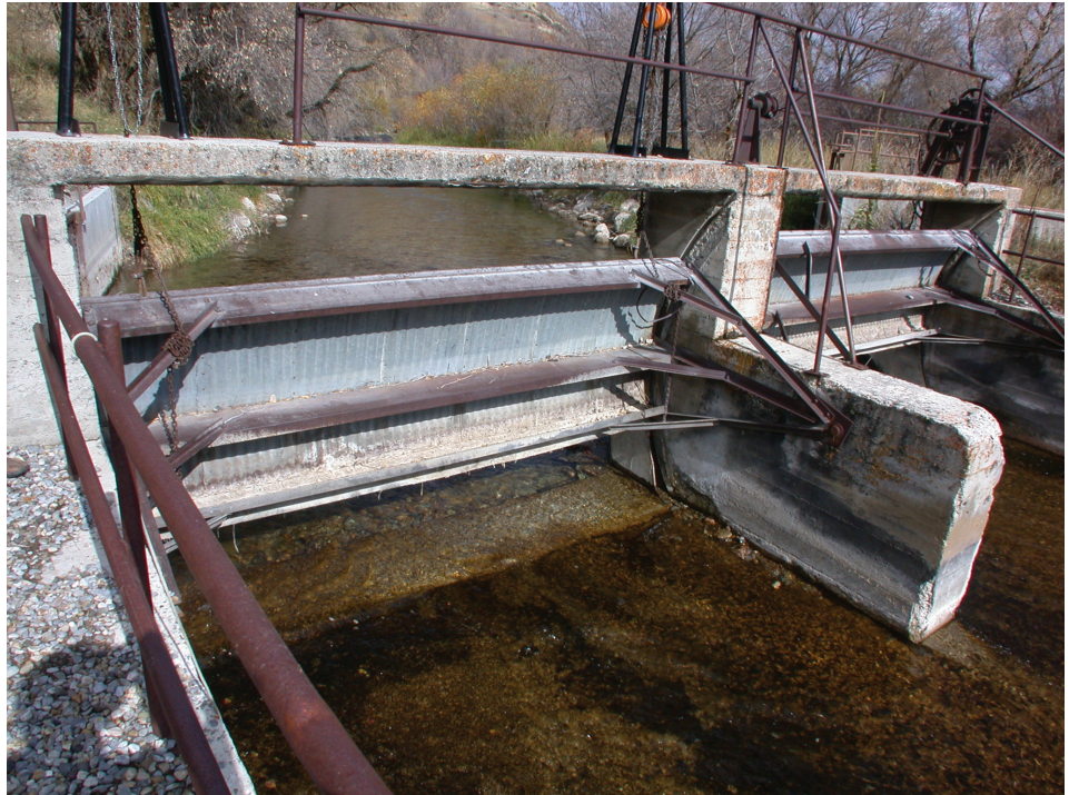
Figure 4.17—Radial gates at lower Cub River diversion, Bear Lake watershed, ID. These gates are open now, but when closed, they raise the upstream water surface elevation by about 2½ feet.
