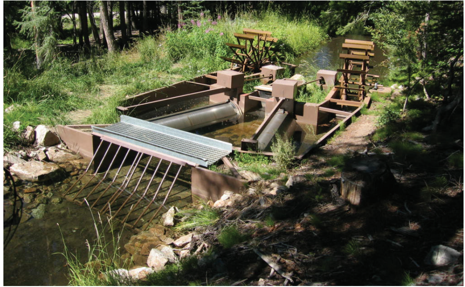
Figure 5.1—Looking downstream at double rotary drum screen installation on Fourth of July Creek diversion, Salmon River Basin, ID.
