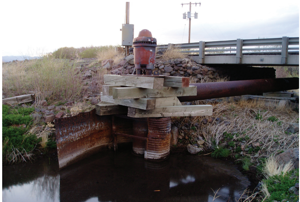
Figure 4.27—Propeller pump installation at Hart Lake, OR.
