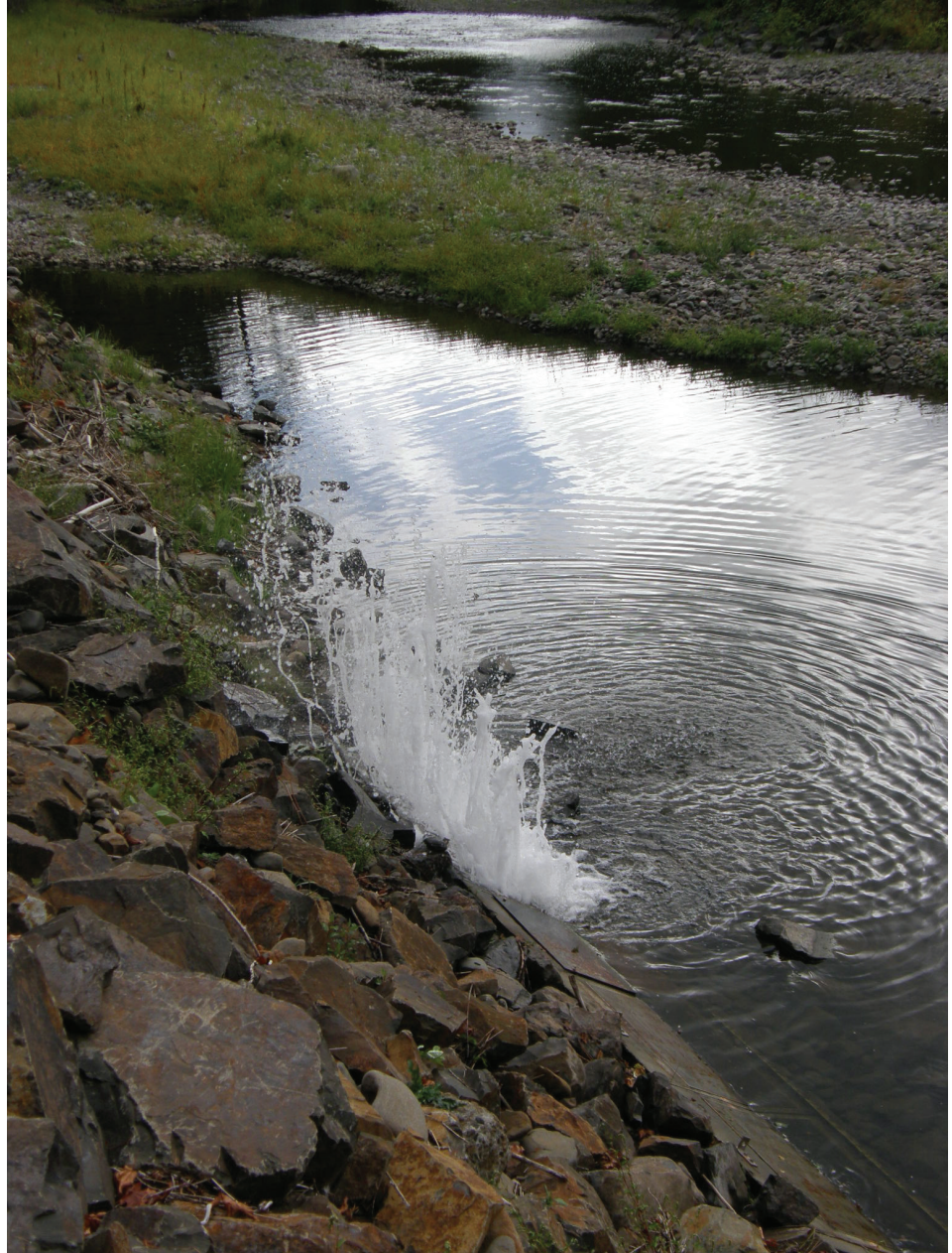
Figure 5.6—Water-burst backwash system operating on one of several screens at bank toe on Kalapuya River, OR. This screen feeds water to a pump sump for the Brownsville municipal water system. This screen also is pictured in figures 4.24 and 4.26.
