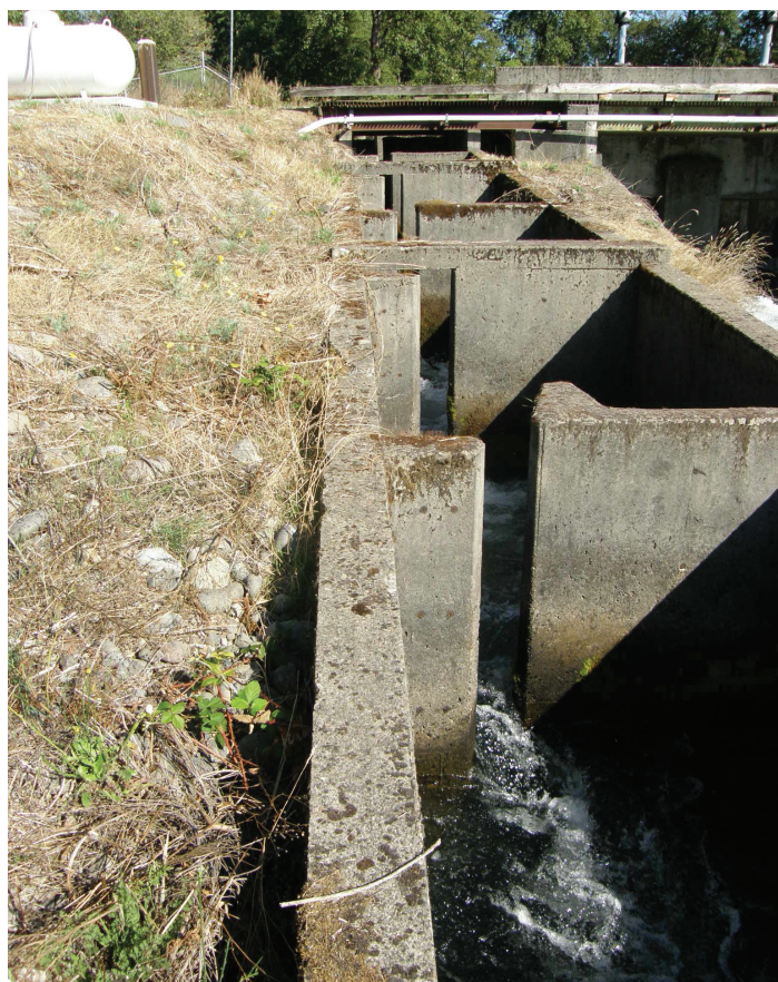
Figure 5.14—Vertical-slot fish ladder, Santiam Water Control District diversion canal, OR.
