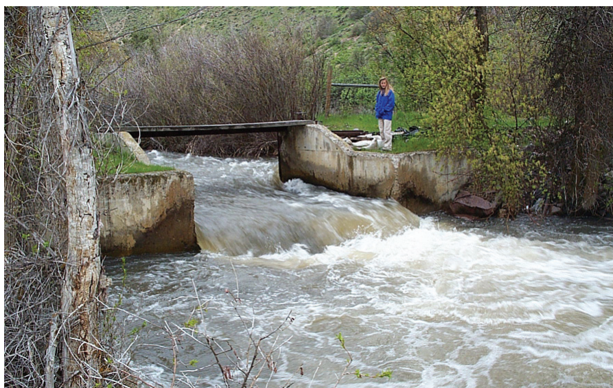
Figure 2.1—Where a permanent diversion structure is narrower than the bankfull channel, flow accelerating across the structure often scours a plunge pool immediately downstream, frequently causing bank erosion and fish passage problems. Cottonwood Creek, ID.
