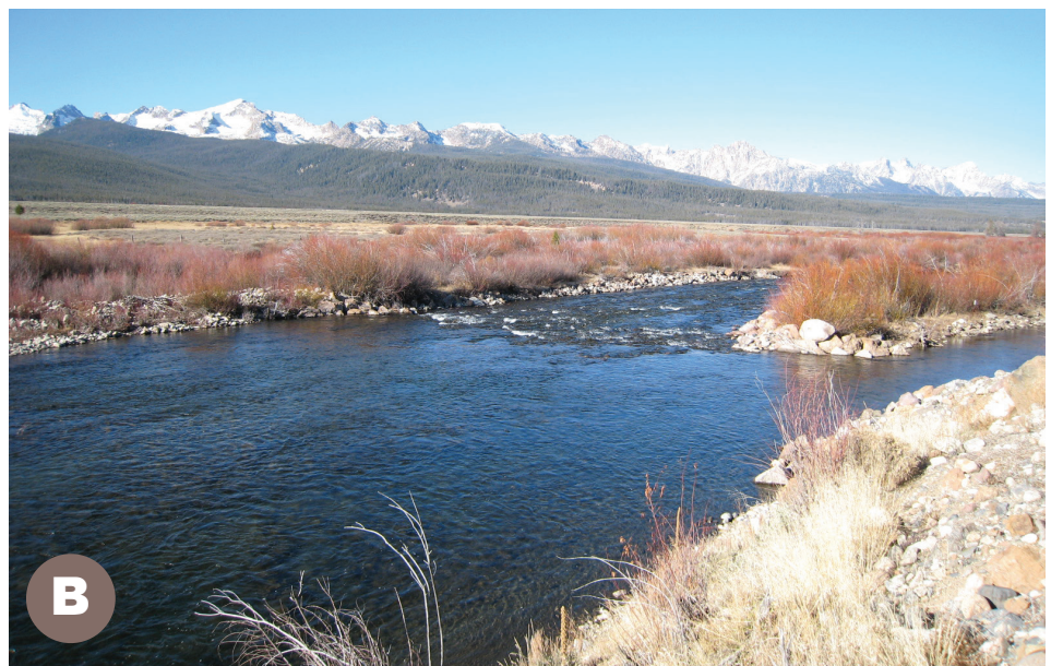
Figure 4.8—(A) Constructed rock riffles on Upper Rock Creek, Bear Lake watershed, WY. (B) Rock ramp—essentially the same as a rock riffle—constructed in 2007 on the Salmon River, ID.
