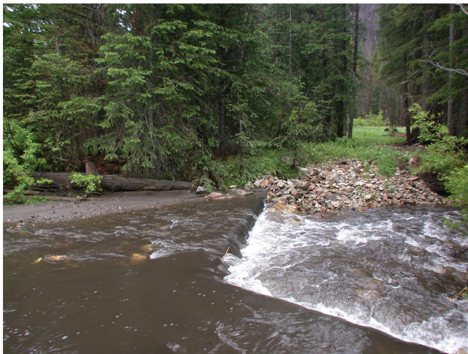
Figure 4.5—Nonadjustable log weir on Fourth of July Creek, Sawtooth National Recreation Area. This watershed burned after the diversion structures were installed. Note that high flows have already begun to outflank the structure.
