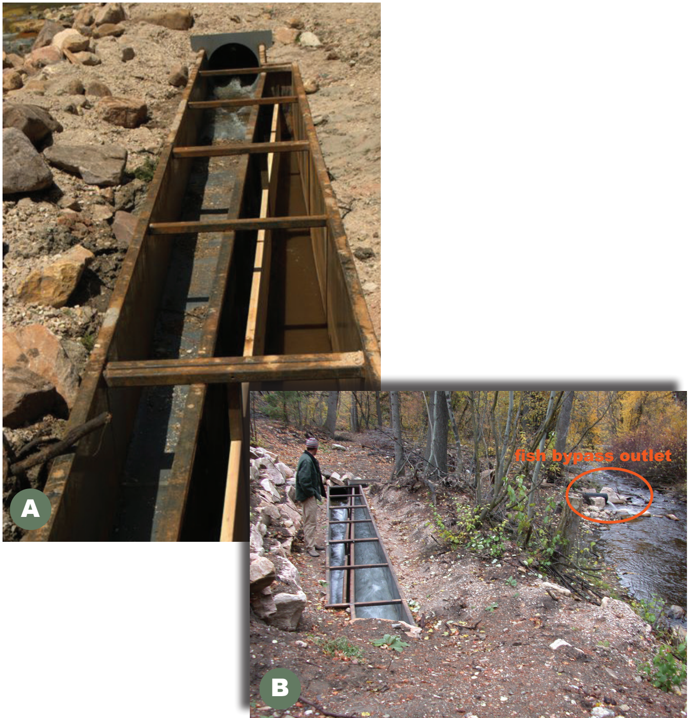
Figure 5.4—Horizontal flat-plate screen. Upper Fish Haven Creek, Bear Lake, ID. (A) Photo was taken during installation. The view is upstream looking toward the headgate. In this Farmers' Conservation Alliance screen, the partially shadowed screen is on the left, with some debris on top. Boards in the middle control how much flow exits toward the diversion ditch, which is out of sight behind the photographer. (B) This view is looking downstream. When the screen is functioning, fish pass over the screen, and out the bypass pipe seen in the background, right. These screens require substantial bypass flow. At least 6 inches of fast-moving water is needed to protect the fish from scraping on the screen, and to sweep the screen of debris.
