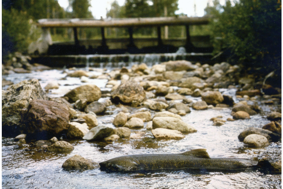
Figure 1.9—This diversion dam was a barrier to upstream passage of fish, including the chinook salmon shown here. The dam has since been removed. Alturas Lake Creek, ID.
