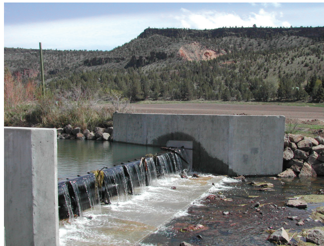
Figure 4.14—Air-bladder diversion dam on Ochoco Creek, OR. A fish ladder is located to the left of the photo. The structure is reinforced at the ends with rock riprap to limit erosion around the concrete wingwalls. Longer wingwalls than shown
