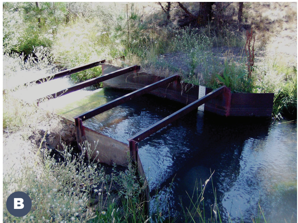
Figure 6.5—Parshall flume (A) drawing. (B) Parshall flume in an unnamed irrigation lateral west of Terrebonne, OR.
