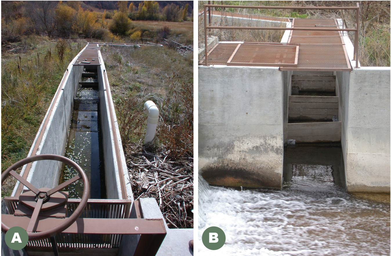
Figure 5.13—Pool-and-weir fish ladder built for spring-spawning Bonneville cutthroat trout, Cub River, tributary of Bear River, ID. (A) General view of the ladder looking downstream. Ladder is nearly dewatered at this time. (B) Looking upstream from the ladder entrance. When the ladder is functioning, the 1-foot weirs are overtopped and water plunges into the pools between them. Note the offset orifices cut into the bottom flashboard, which permit whitefish to swim through and rest in eddies behind the weirs. This ladder serves the diversion dam pictured in figure 4.3; its concrete wall is visible in the center-right of that picture.
