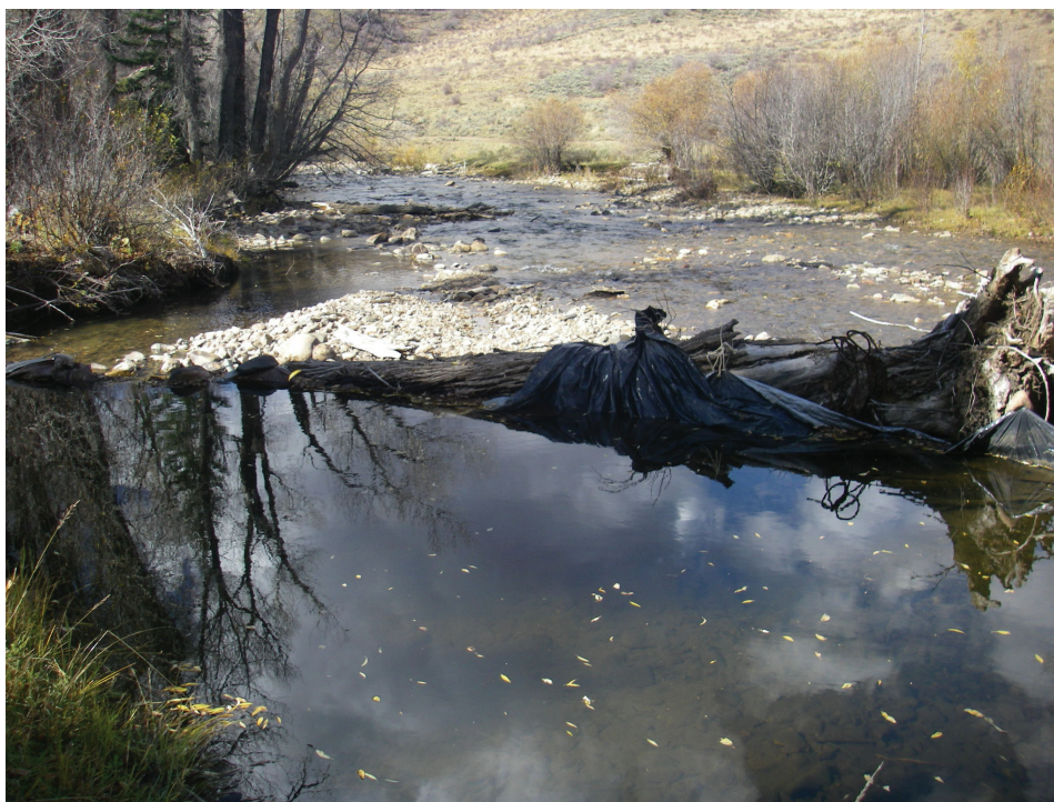
Figure 4.18—Check structure using logs to support a plastic tarp on the Medicine Bow National Forest, WY. The ditch is to the left out of the photo. This check structure is not removed at the end of the season.
