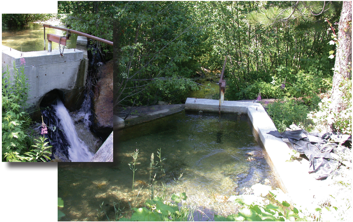
Figure 1.4—Concrete diversion dam on Archie Creek, Boise National Forest, ID. The substantial (approximately 5 foot) downcutting caused by the dam on this small, steep stream can be seen beyond the dam in the distance, and in the inset. Plastic sheeting seen on the right bank is a temporary fix for the soil piping that, if left unchecked, will undermine the dam.
