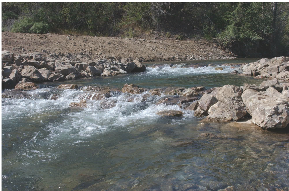
Figure 4.20—Bulldozer-constructed wingdam with diverted water in foreground. East Fork Salmon River, ID. This diversion was replaced and combined with another diversion in a Bureau of Reclamation project aimed at reducing harm to anadromous and resident fish species in 2003. Photo courtesy of Brian Hamilton, Bureau of Reclamation, Salmon, ID.
