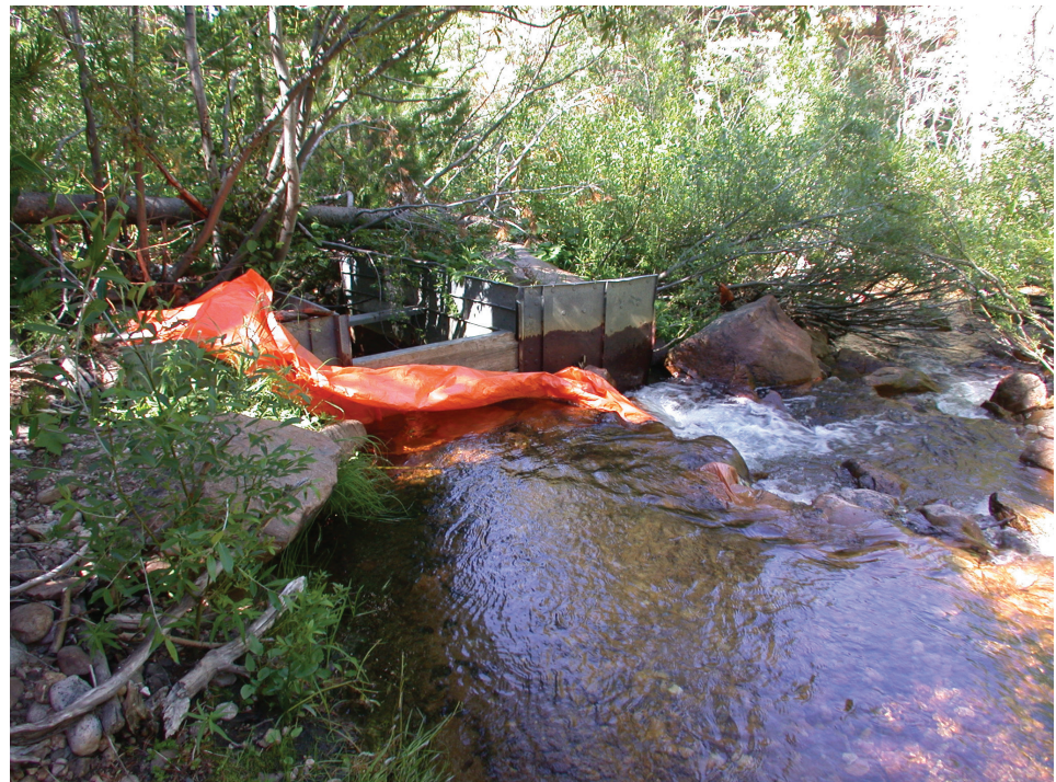
Figure 3.8—Stoplog weir headgate on Soldier Creek, Medicine Bow National Forest, North Platte watershed, WY. The plastic sheeting indicates the problem occurring with leakage through and under the closed headgate. To the right is a rock weir check structure.
