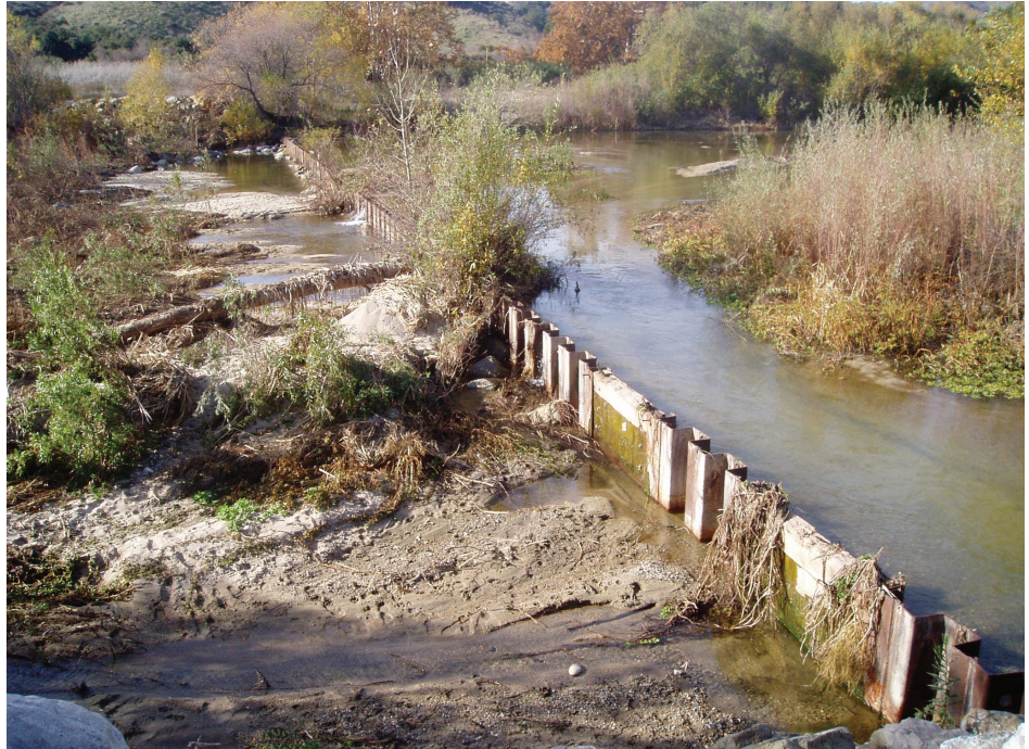
Figure 1.3—Santa Margarita River O’Neil diversion weir at Camp Pendleton, CA. This steel pile dam is in a river with very high sediment load. Heavily vegetated sediment accumulations upstream and downstream are visible in this photo, which was taken shortly after a moderate flood had disturbed the channel. Photo by Kathleen Frizel, Bureau of Reclamation.
