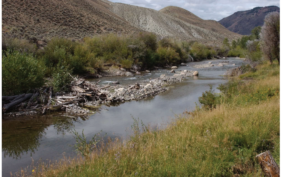
Figure 4.21—Two diversions, including the pushup dam in figure 4.20, were consolidated into one on the East Fork Salmon River. The new diversion structure is an A-weir with two rock weir drop structures for salmonid fish passage. Photo courtesy of Brian Hamilton, Bureau of Reclamation, Salmon, ID.
