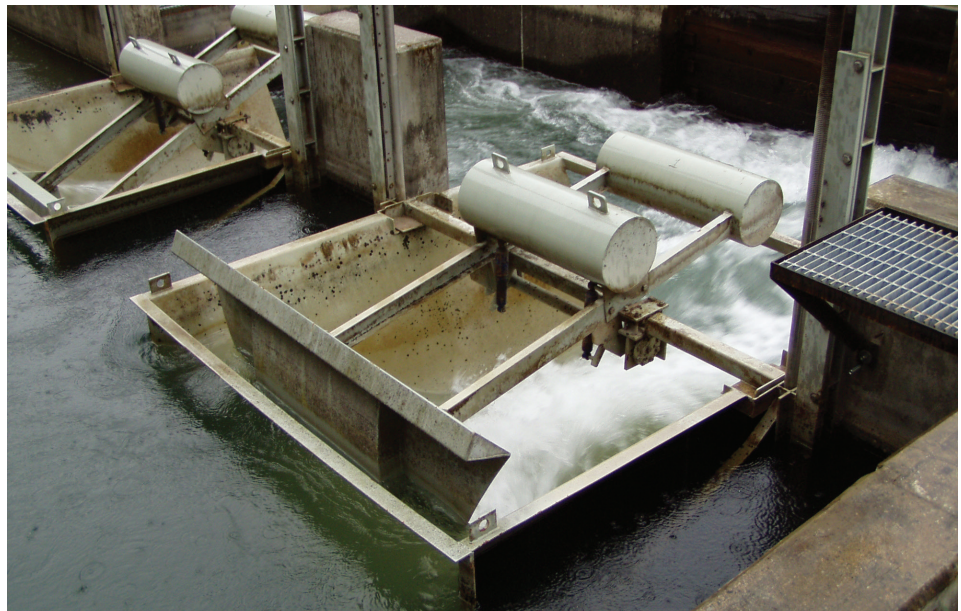
Figure B.1—Automatic float gate used to maintain constant water level on the inlet screen for the Hood River Canal Diversion, Hood River, OR. Only the closer gate is operating, and it is adjusting to keep the upstream (on left) water level the same. The float or ballast is the round tube at the end of the levered gate.
