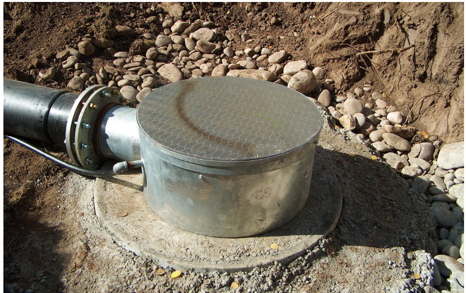
Figure 5.3—Pressure backwash flat plate fish screen at the end of a pump suction. This intake is in a channel undergoing reconstruction after an impoundment was removed. Garden Creek, Bonneville County, ID. Photo courtesy of Matt Woodard, Trout Unlimited.
