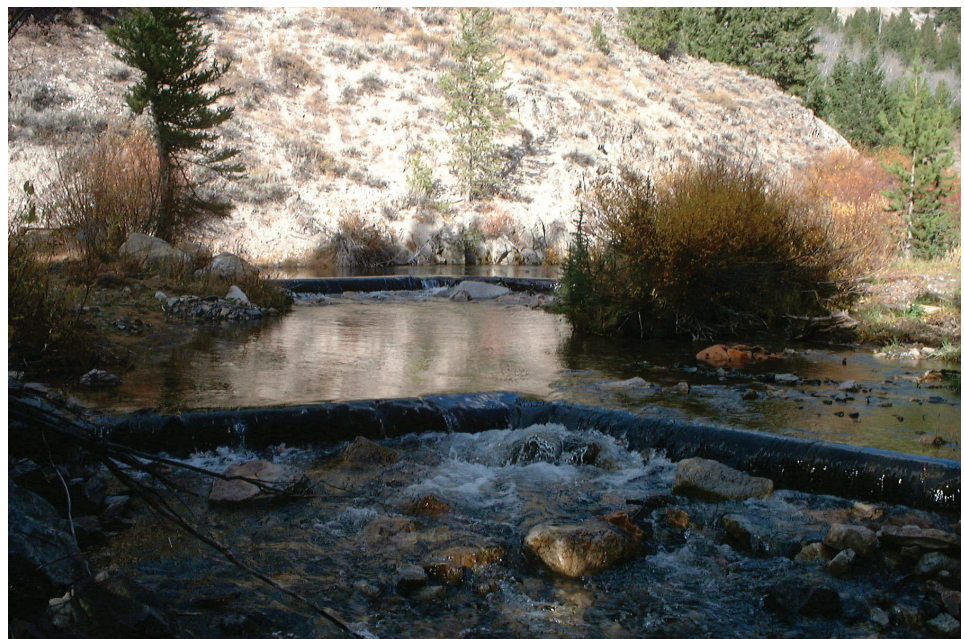
Figure 4.10—Two log weirs installed as diversion checks on Fourth of July Creek, Sawtooth National Recreation Area, ID. This is the same installation pictured in figure 4.5.
