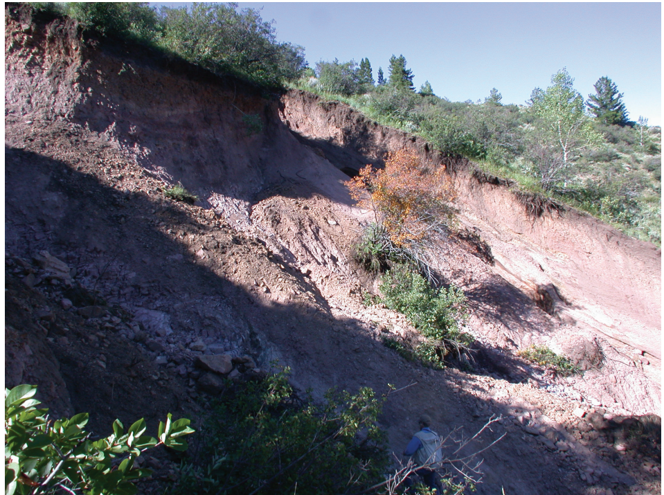
Figure 1.8—Massive slope failure along diversion ditch. The failure was caused by poorly controlled flows at the headgate and debris accumulation in ditch, causing the ditch berm to fail by overtopping or percolation through root or small animal holes. Soldier Creek, Medicine Bow National Forest, WY. Figure 3.8 shows the headgate.
