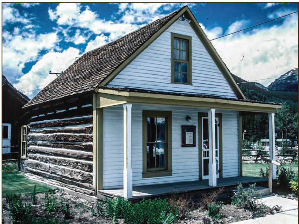
Figure 27—This log cabin in Frisco, CO, has clapboard siding on the front.
