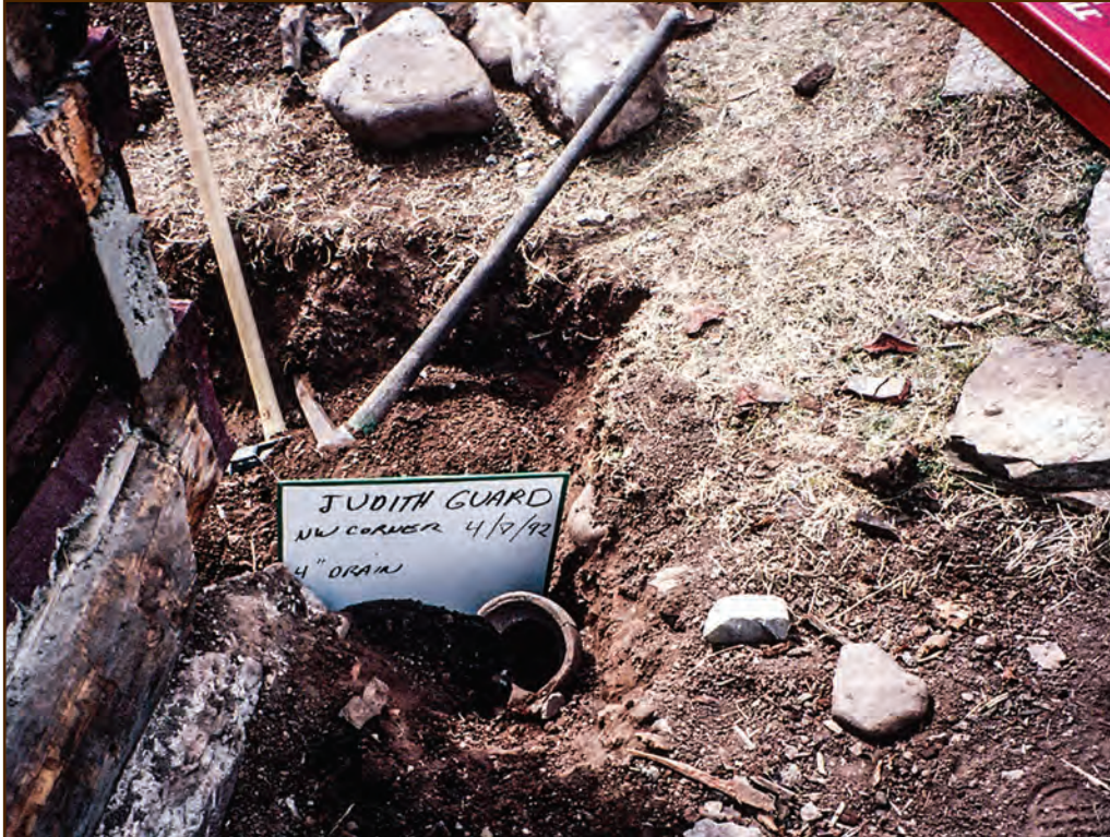
Figure 2—The photographer made and placed a signboard in this photo to show that the circular fragment is a 4-inch-diameter drain tile found during a restoration project on April 8, 1992, at the northwest corner of the Judith Guard Station (Lewis and Clark National Forest, Northern Region). Sign boards in photos, unlike other photo captions, can't be separated and lost from the photo.
