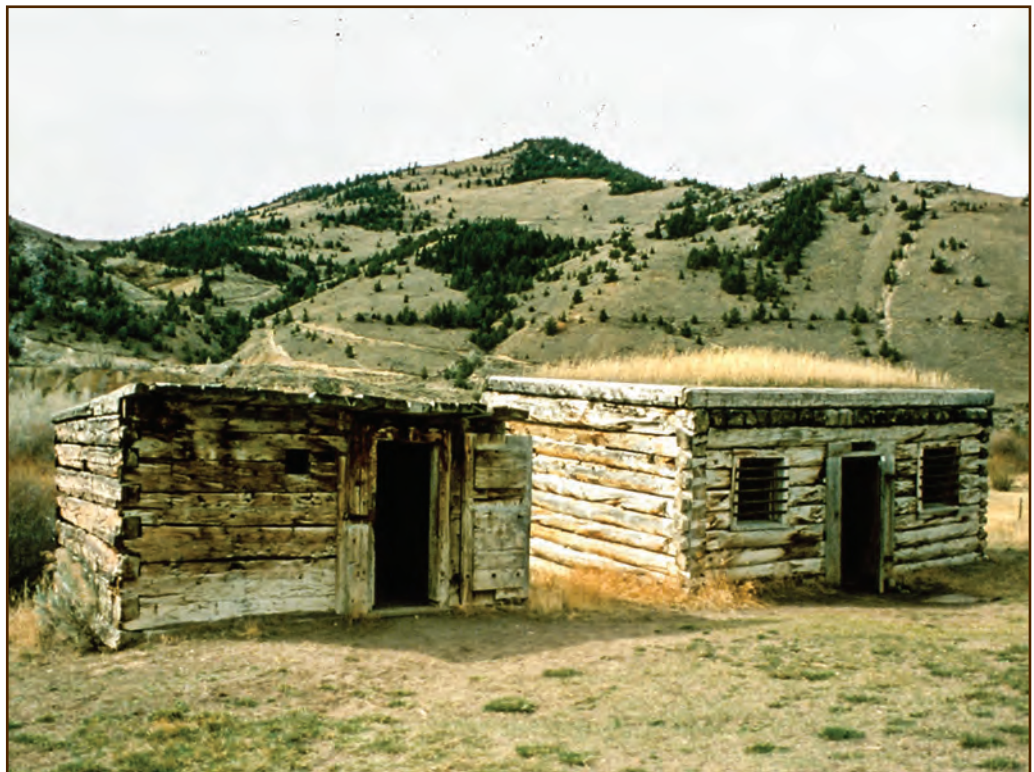
Figure 29—These historic log jail buildings at Bannack State Park in Montana have sod roofs.
