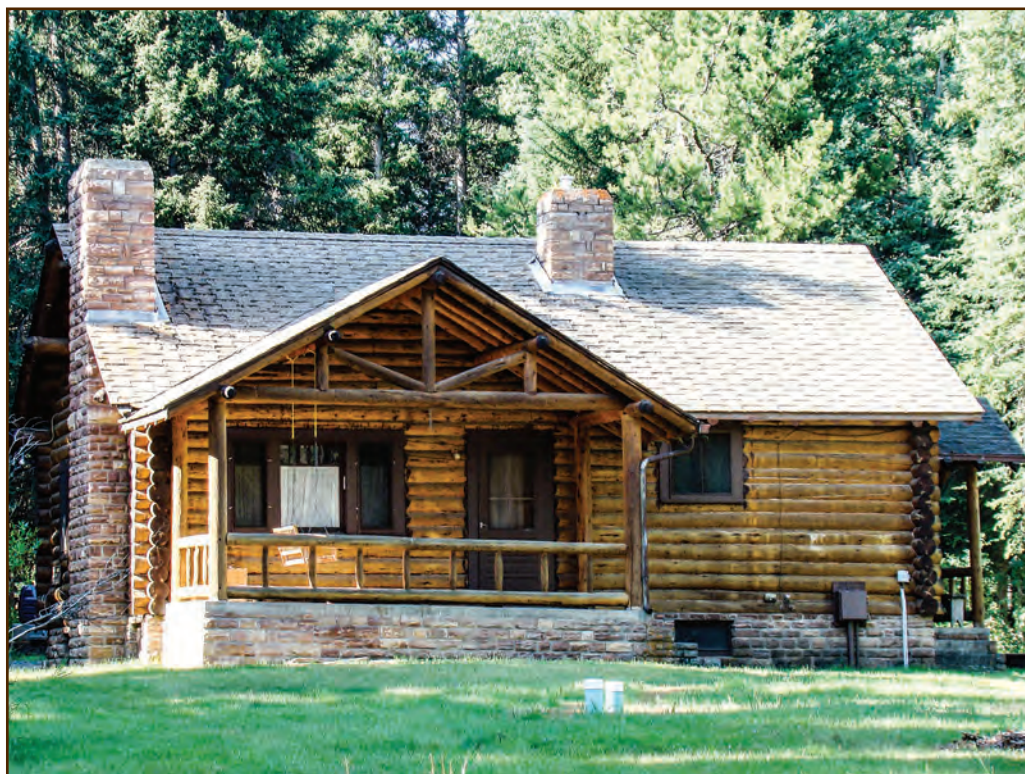
Figure 9—The Ranger’s House at the Crandall Ranger Station (Shoshone National Forest, Rocky Mountain Region), built in 1935, has a mortared stone foundation.
