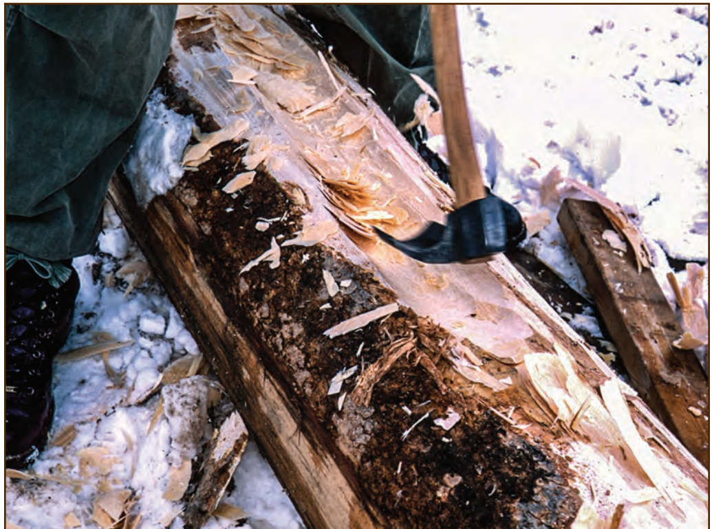
Figure 114—Secure the log upside down on the ground when you use an adz to create a cope.
