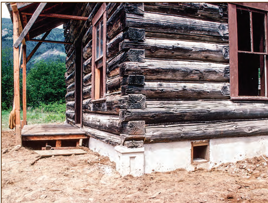
Figure 86—The completed replacement foundation matches the appearance of the original foundation, including the forming details on the corners. Preservation crewmembers created foundation vents out of the gaps in the foundation through which the steel beam needles extended.
