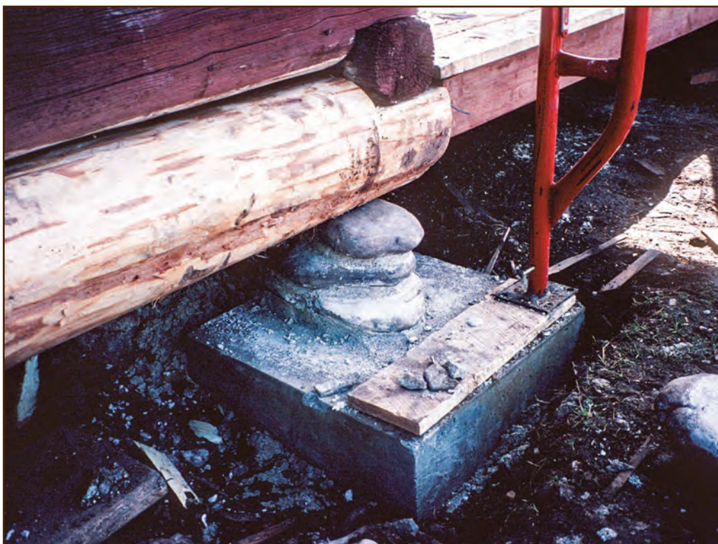
Figure 81—Preservation crewmembers constructed a new footing and stone pier at the Judith Guard Station of the Lewis and Clark National Forest, Northern Region. The footing is under a corner of the cabin where the wall meets the porch.
