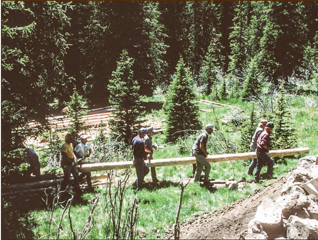
Figure 110—This eight-person crew can safely and easily move a large log.
