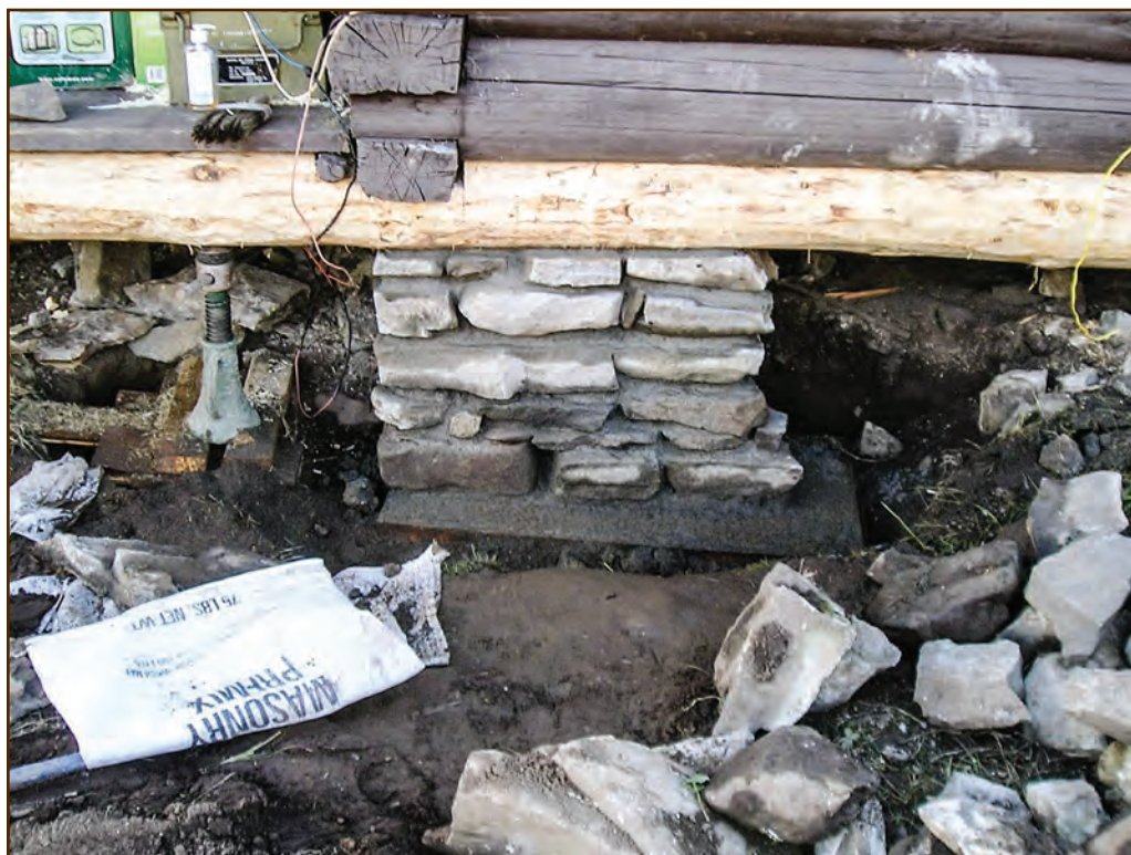
Figure 82— A preservation crewmember constructed a new footing and sturdy flat stone pier at the Badger Cabin within the Lewis and Clark National Forest, Northern Region.
