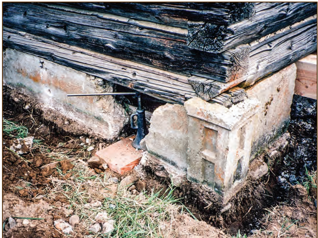
Figure 84—Preservation crewmembers removed part of the foundation to allow placement of a jack (center) and a timber needle (far right) to support the cabin during foundation removal and log replacement. The crewmembers replaced these temporary supports with steel needles on cribbing before forming the new foundation.
