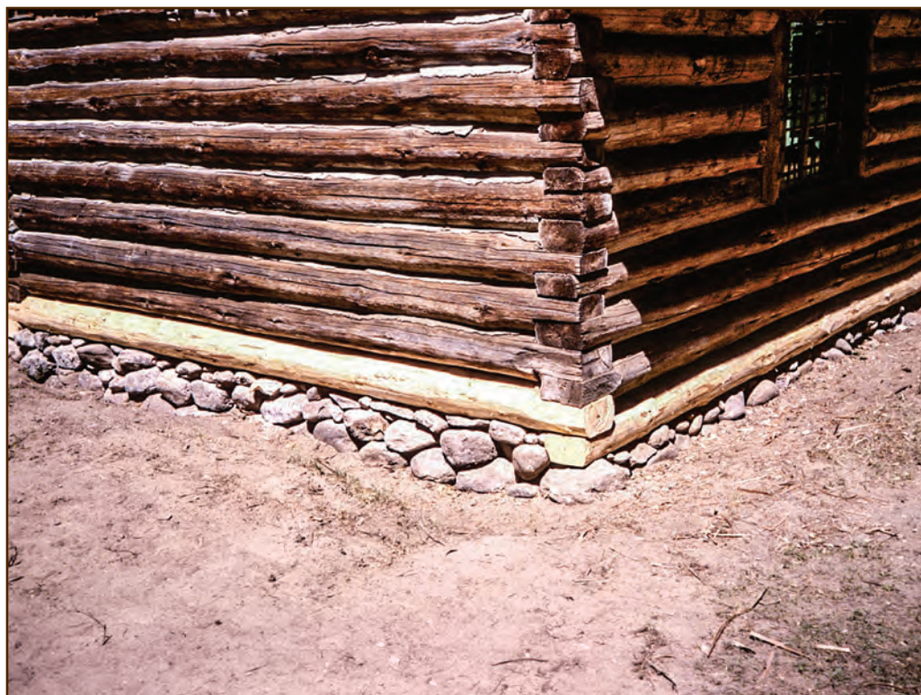
Figure 87—Preservation crewmembers constructed a new cobblestone foundation under the Cooper's Flat Cabin in the Bitterroot National Forest, Northern Region.
