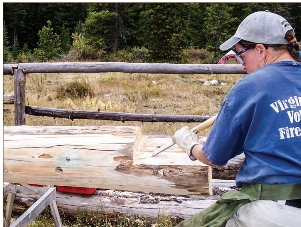
Figure 112—The author uses a chisel to shape the end of a log for the cabin at Badger Station of the Lewis and Clark National Forest, Northern Region.
