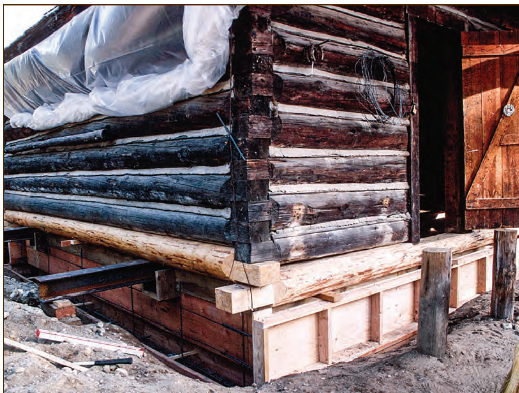
Figure 85—Preservation crewmembers replaced deteriorated logs and constructed forming for the new foundation around the steel beam needles that support this cabin.
