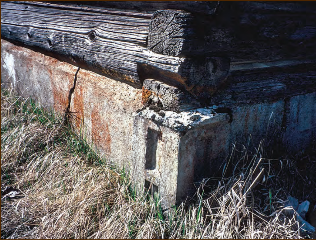
Figure 83—This foundation corner is cracked and leans out, but it's more intact than the rest of the foundation under the Bull River Guard Station of the Kootenai National Forest, Northern Region. The forming details in the concrete are important to the appearance of the building.
