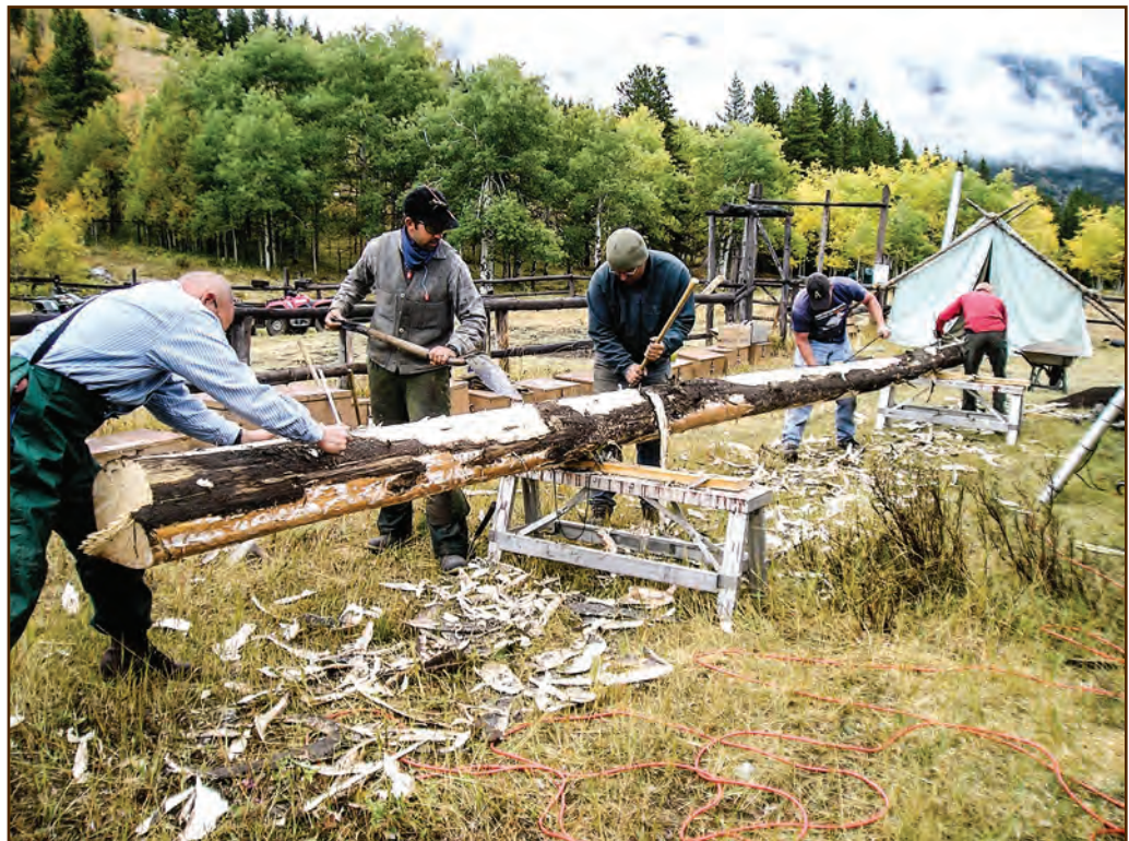
Figure 111—This crew used drawknives, shovels, and a bark spud to remove the bark from a replacement log for the cabin at Badger Station of the Lewis and Clark National Forest, Northern Region.
