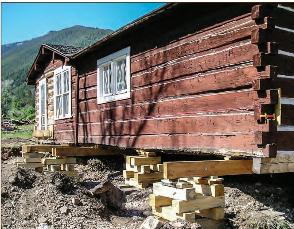
Figure 76—Preservation carpenters raised the Sage Creek Cabin (Custer National Forest, Northern Region) 18 inches during a 2-week period, using needles, jacks, and cribbing.
