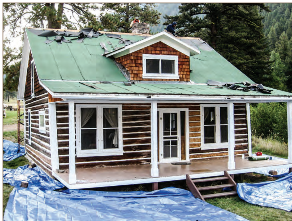
Figure 282—These roofers are replacing the old asphalt rolled roofing at Hogback Cabin (Lolo National Forest, Northern Region). The roofing had deteriorated along the unusual vertical seams. Roofers usually lay asphalt rolled roofing with horizontal seams.
