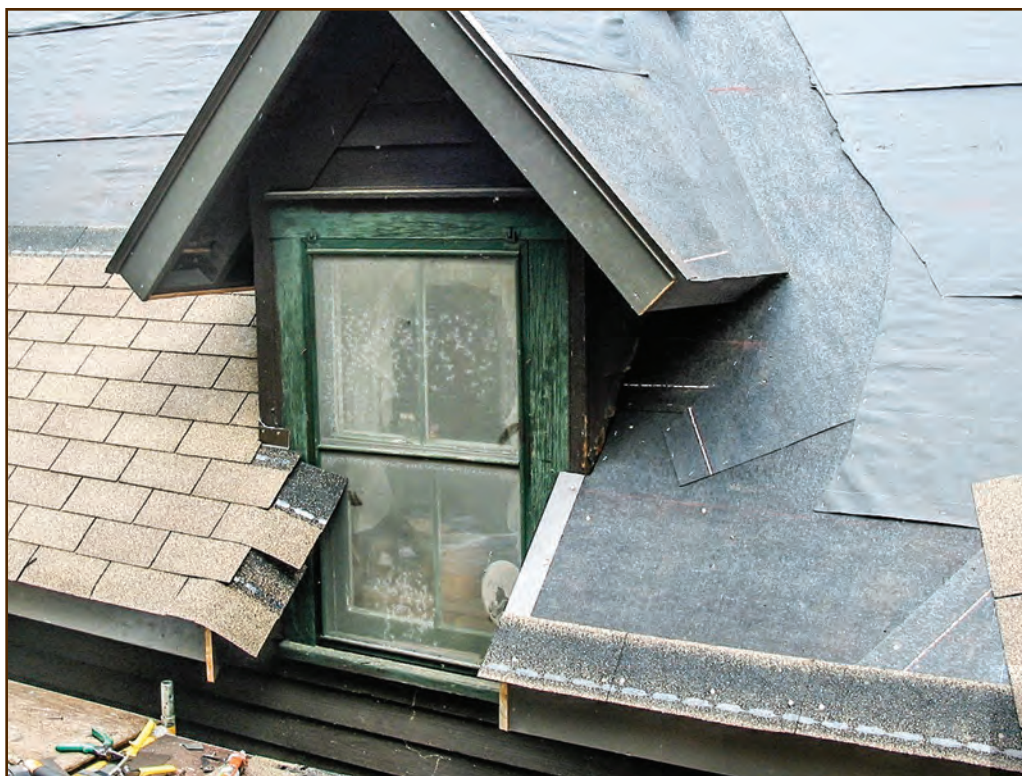
Figure 284—As shown in the lower right of this photo, roofers created an asphalt shingle starter course for the roof of this historic log cabin by cutting the tabs off regular shingles. Note the position of the adhesive spots near the eave edge of the shingles. The original builders constructed the log part of the cabin, known as “the Homestead,” in the early 1800s on what is now the Bradford District (Allegheny National Forest, Eastern Region). The owner added frame wings in the early 1900s.
