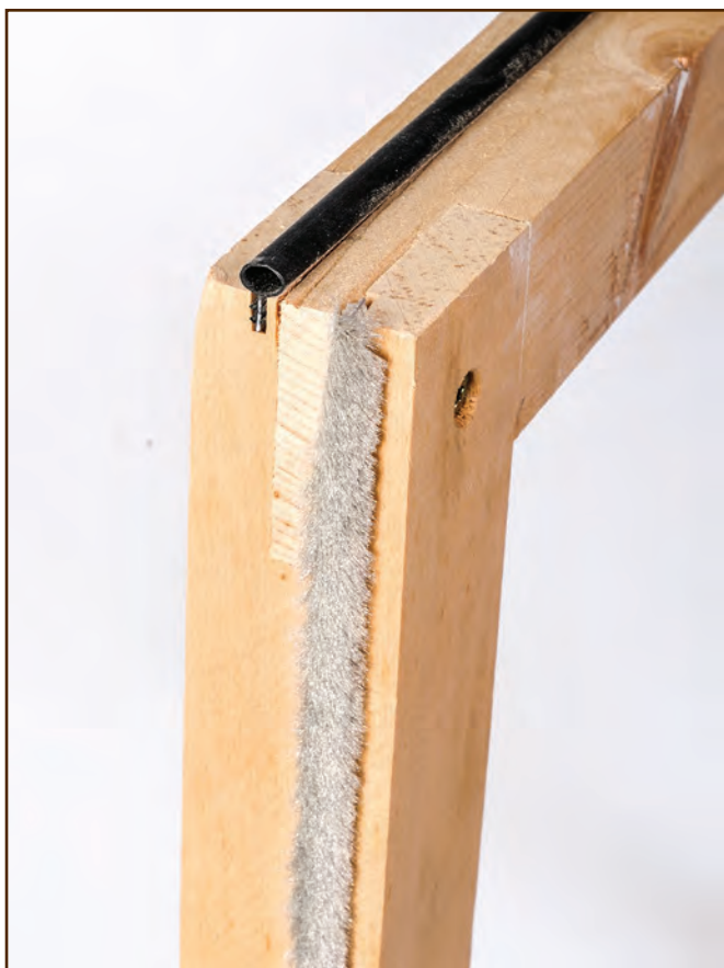
Figure 302—This mock-up of a small double-hung window shows bulb-type weather stripping on the top and brush-type weather stripping on the side. Notice how the flanges on the weather stripping fit into routed slots in the frame and hold the weather stripping in place without fasteners.
