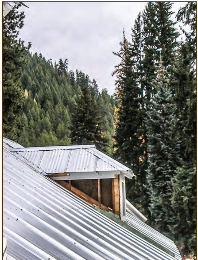
Figure 281—The ridge cap is the final element that you install on a metal roof. In this photo, the roof is complete, but the preservation crew has not yet replaced the siding on the dormer.
