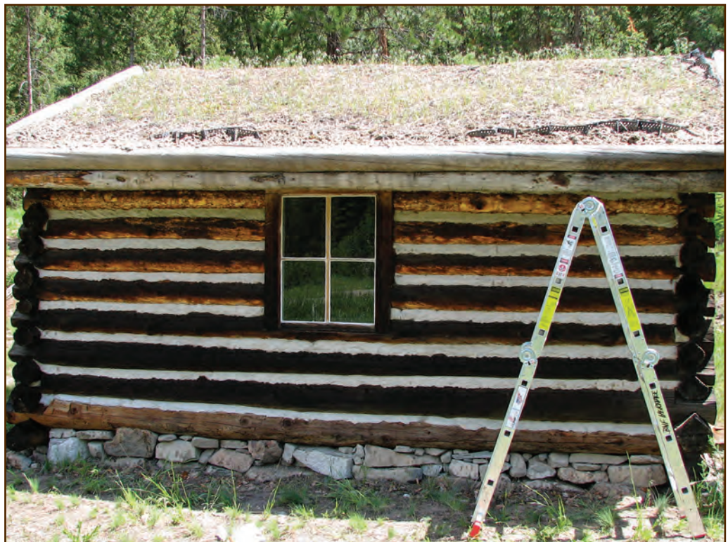
Figure 289—When preservation crewmembers replaced the sod roof of the Alta Ranger Station, they put down a layer of ethylene propylene diene terpolymer (EPDM) over the puncheon sheathing, then laid geocell to hold the soil in place. Unfortunately, the crew had to remove the geocell fabric after it warped and emerged from the soil.
