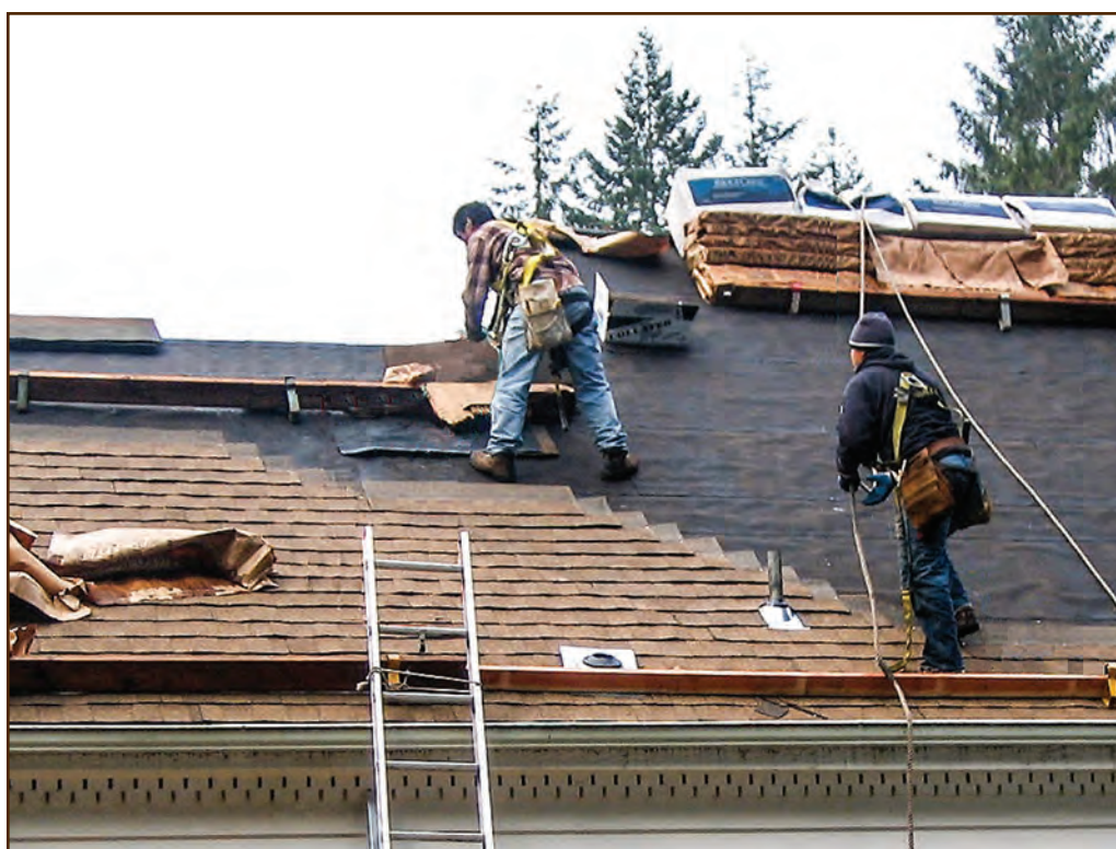
Figure 285—When the roofers replaced the roof on this 1936 residence, they applied asphalt shingles in a stair step pattern. Roofing nails are visible near the right edge of each tier of shingles. The building, located just north of Lincoln City, OR, is part of the Pacific Northwest Research Station's Cascade Head Experimental Forest.
