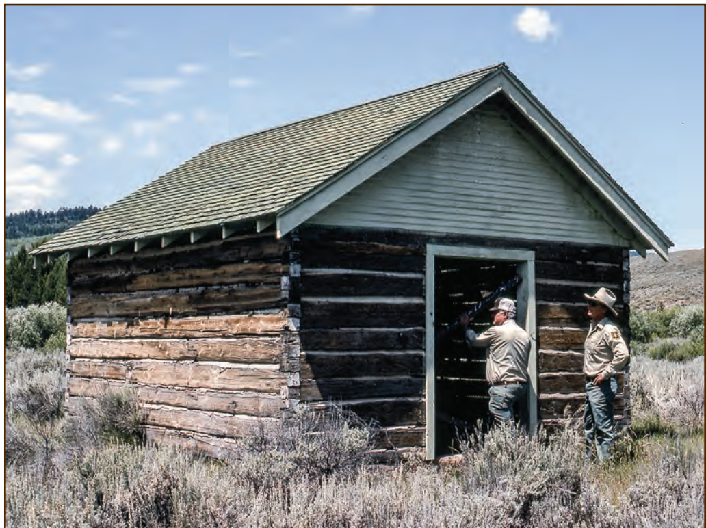
Figure 296—The roof of the 1934 Stump Creek Guard Station fly shed (Caribou-Targhee National Forest, Intermountain Region) still shows the original green roof stain and white trim. A Forest Service crew used logs salvaged from the 1909 Stump Creek Ranger Station buildings to build the shed.
