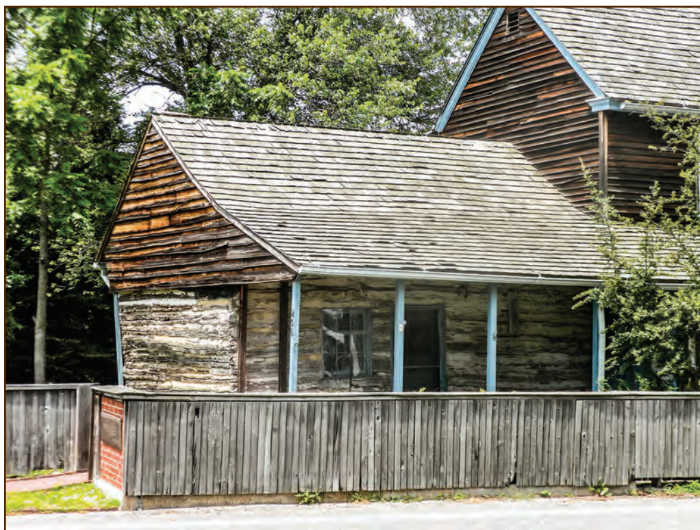
Figure 290—The Nothnagle Log House in Gibbstown, NJ, built around 1638, may be the oldest surviving log cabin in the United States. The original hewn-log cabin is 16 by 22 feet, with full dovetail notching, local clay daubing, and a brick fireplace in one corner. The owner constructed the two-story frame addition in the early 1700s. The building still serves as a home.
