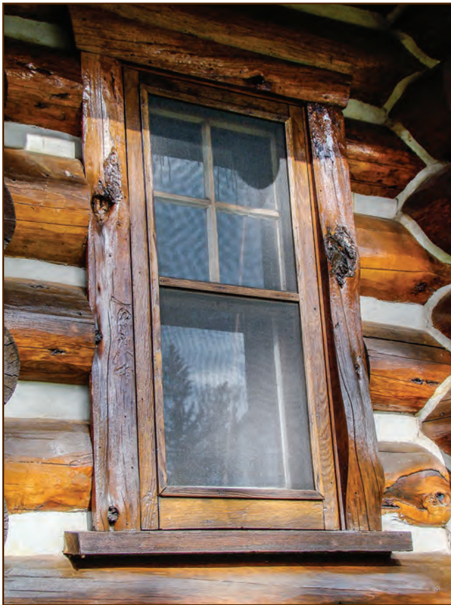
Figure 298—This screened, double-hung window is on a Wyoming Game and Fish cabin at the Sunlight Basin work center. The Sunlight Basin Ranch, established in 1896, included a dude ranch component beginning in 1913. The State of Wyoming acquired the ranch in the mid-1900s.
