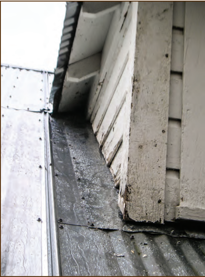
Figure 280—For metal roofing, it is very important for the overlapping lip of each panel to sit properly in the receiving channel of the adjacent panel, as shown on this vertical joint.
