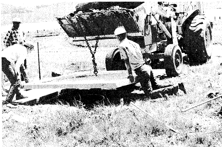
Figure 1.--Installing precast concrete toilet pads.
