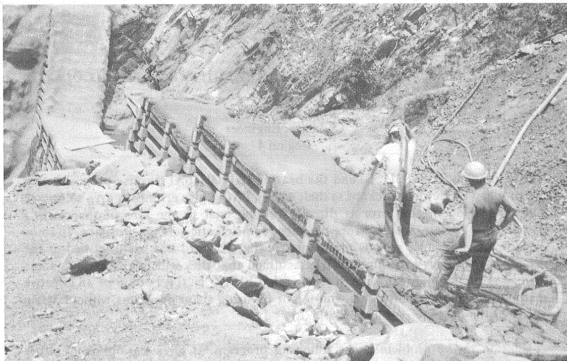
Figure 15. — Guniting top of dam.
