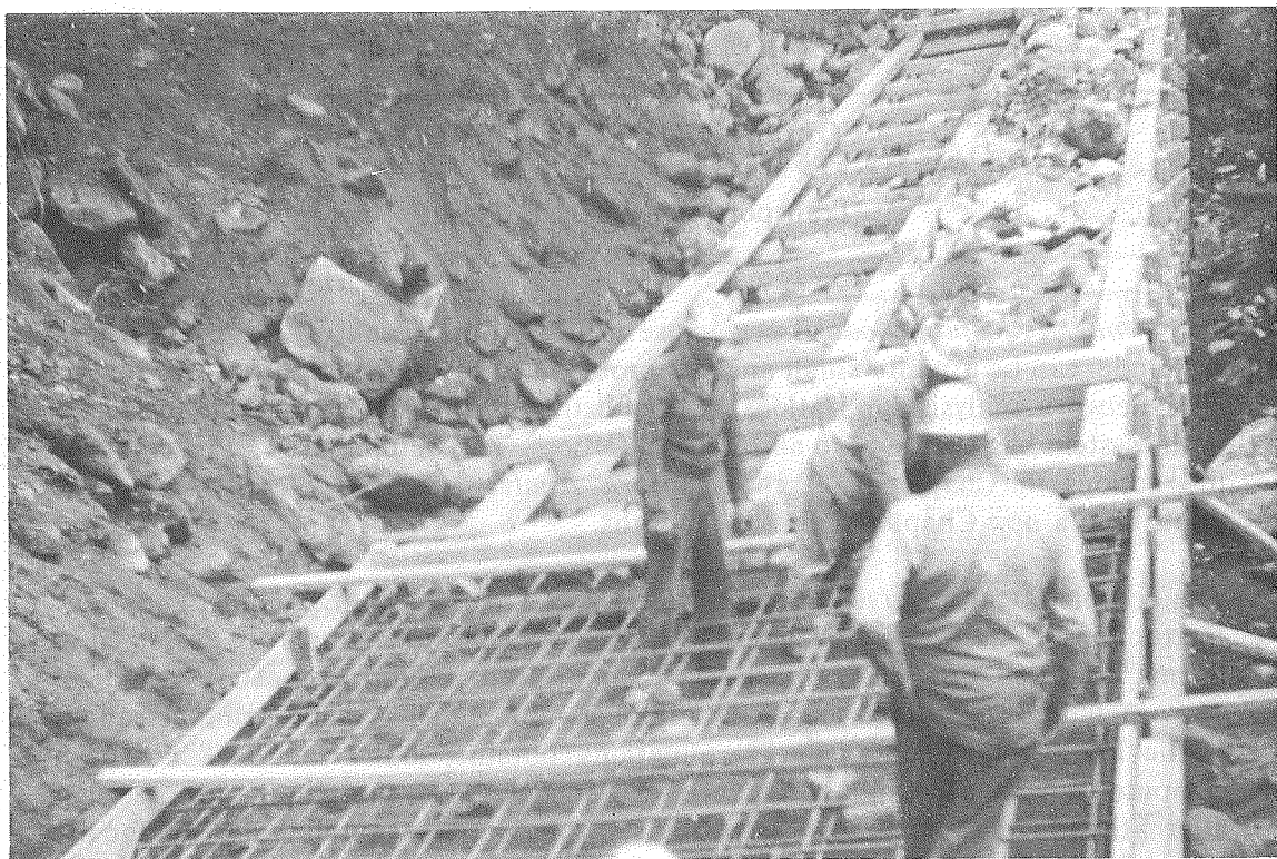
Figure 14. — Construction of step slab.
