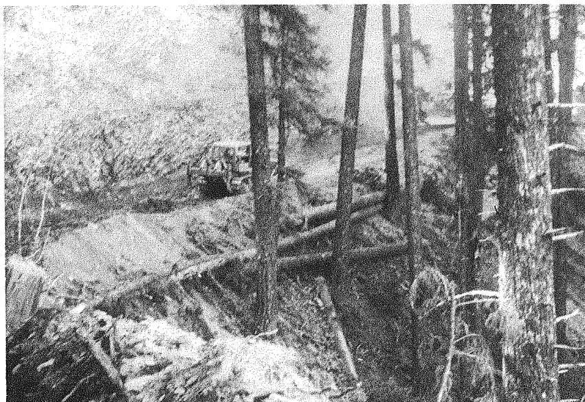
Figure 2. — Barrier trees in place during excavation operation.
