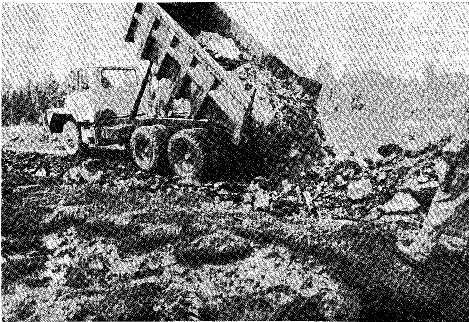
Figure 3. End dumping pit-run rock. The area shown illustrates the results of a typical bearing capacity failure. Severe subsidence of the road embankment and upheaval of the adjacent muskeg occurred immediately. Note the lack of water on the unvegetated muskeg in the foreground; that bare area had about 6 inches of groundwater covering it immediately prior to end dumping.
