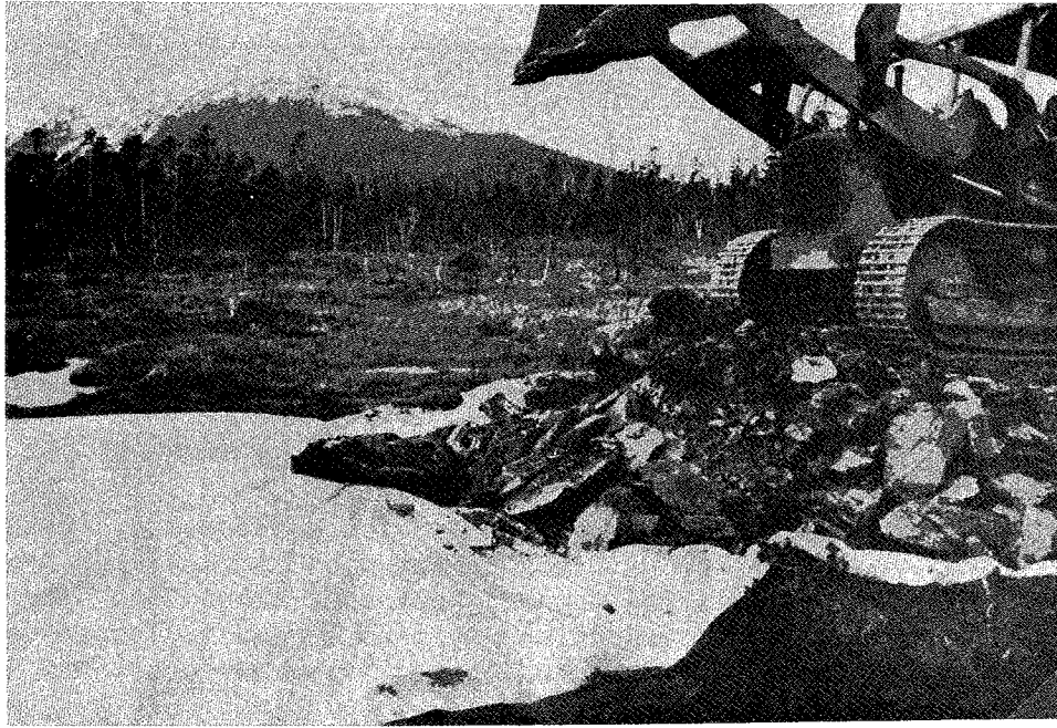
Figure 4. Spreading the pit-run rock.
