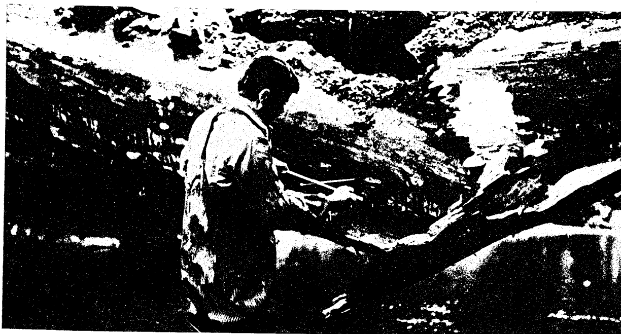
Figure 6 (R-10). Broken stringer log had previously seen service as a spar tree.
