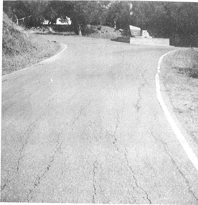
Figure 1. Alligator cracks in 2-1/2 mile road.
