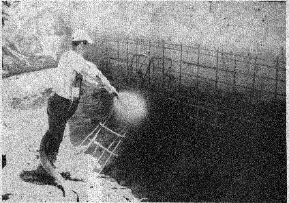
The shotcrete is applied to the downstream side of the structure, covering the rebar framing. Buttresses have been left temporarily through which stream flow can pass.
