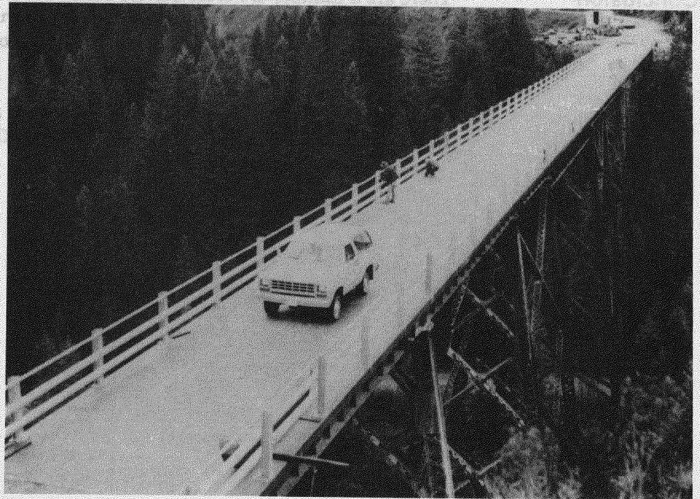
Figure 8.—Structural tube guardrail system being aligned on the Squaw Creek Bridge structure.
