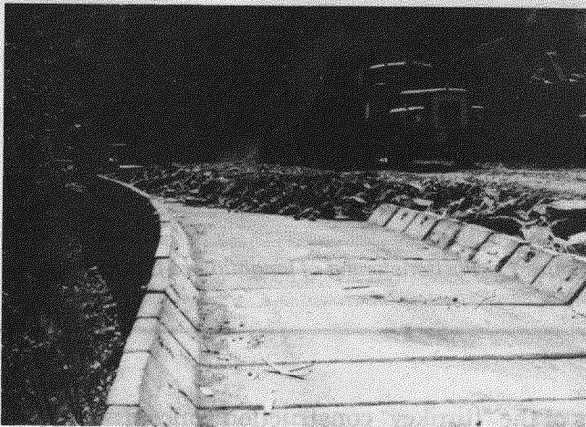
Figure 4.—Construction of the three-tiered retaining wall using the concrete ballast boxes (left) and the completed wall (right).
