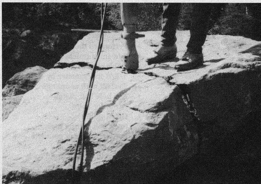
Figure 3.—Split rock—directional breakage, no fly rock, and no spalls.
