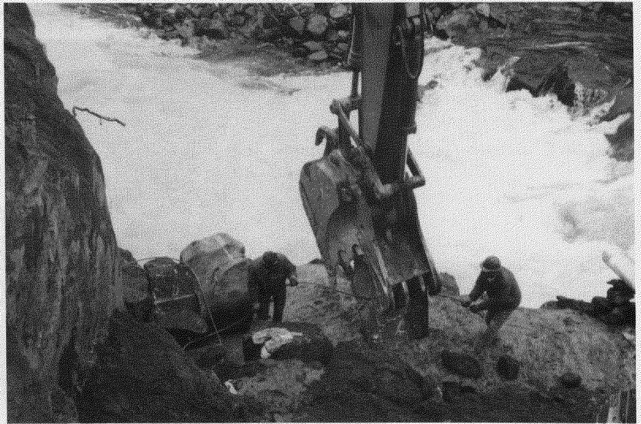
Figure 4.—Excavator holds necklace block, crew threads cable.
