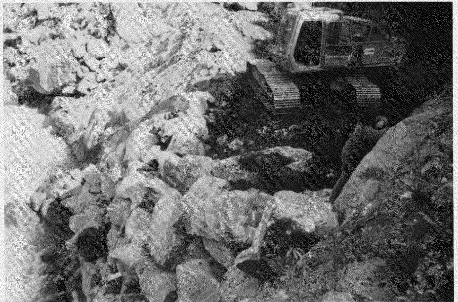
Figure 8.—Placing top portion of riprap above necklace wall.
