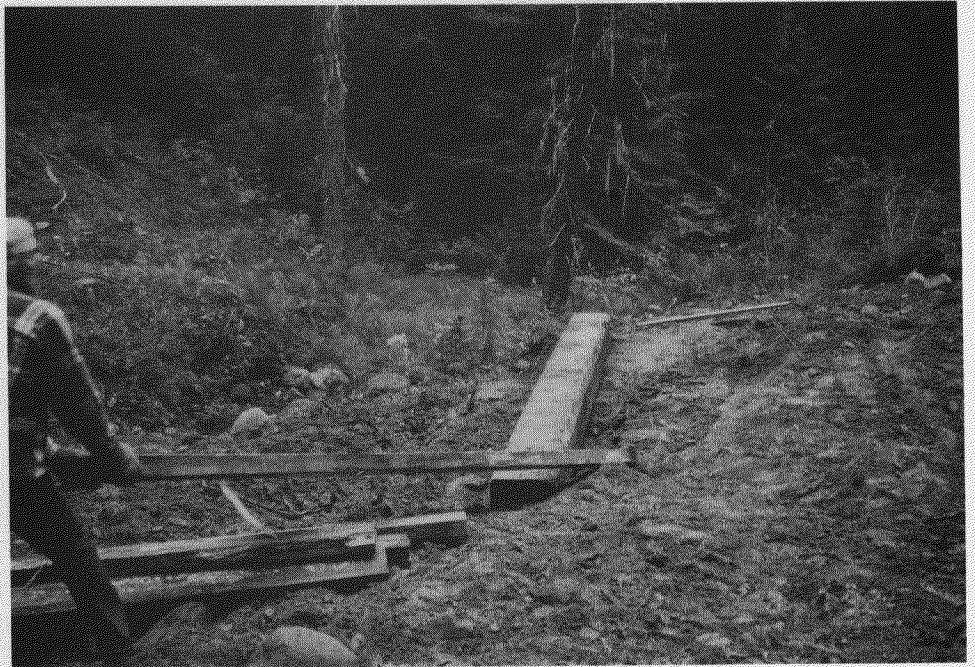
Figure 6.—Placement of sill timber prior to bridge placement.
