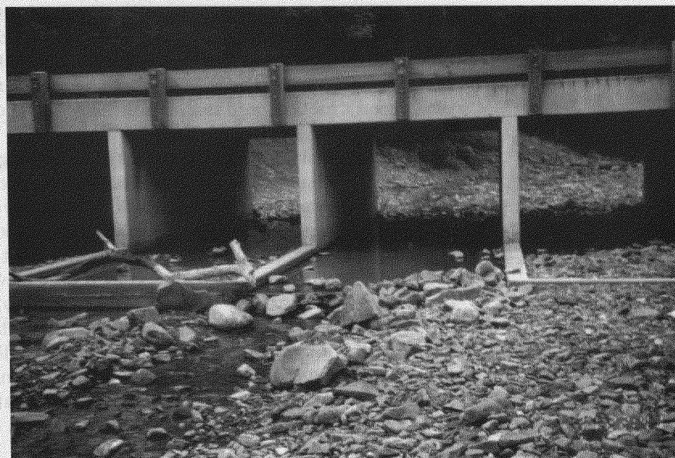
Figure 3.— Low flow concentrated in the uncurbed outlet.
