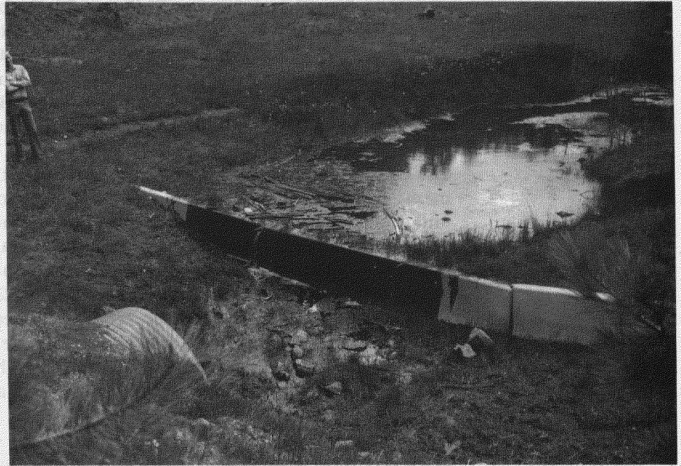
Figure 7.—Jersey barrier gully plug.
