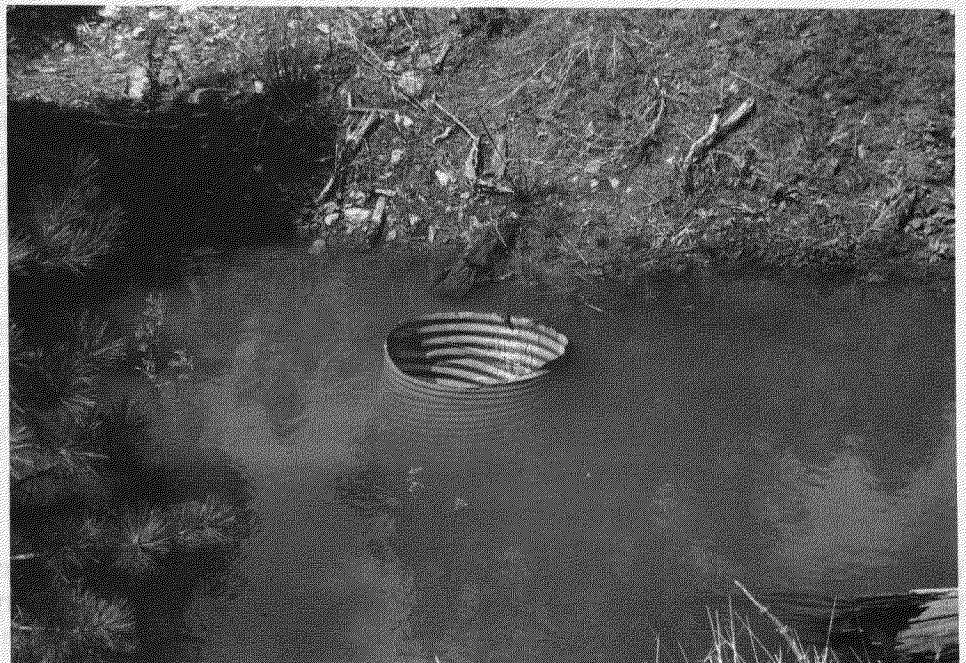
Figure 4.—Elbow installed on cross drain to pond water and preserve sediment.
