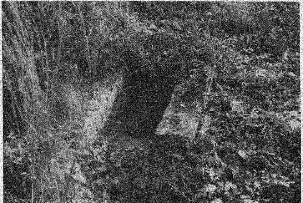
Figure 12.— Self-cleaning catch basin constructed by the CCC.
