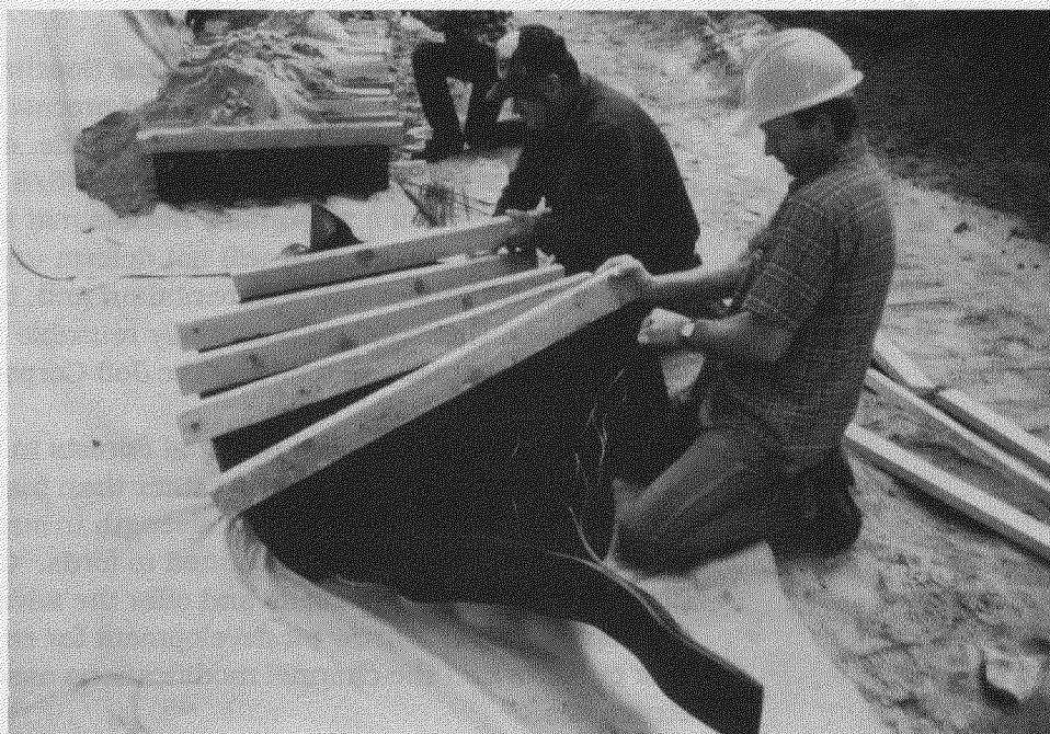
Figure 10.—Expanding confinement cell units.
