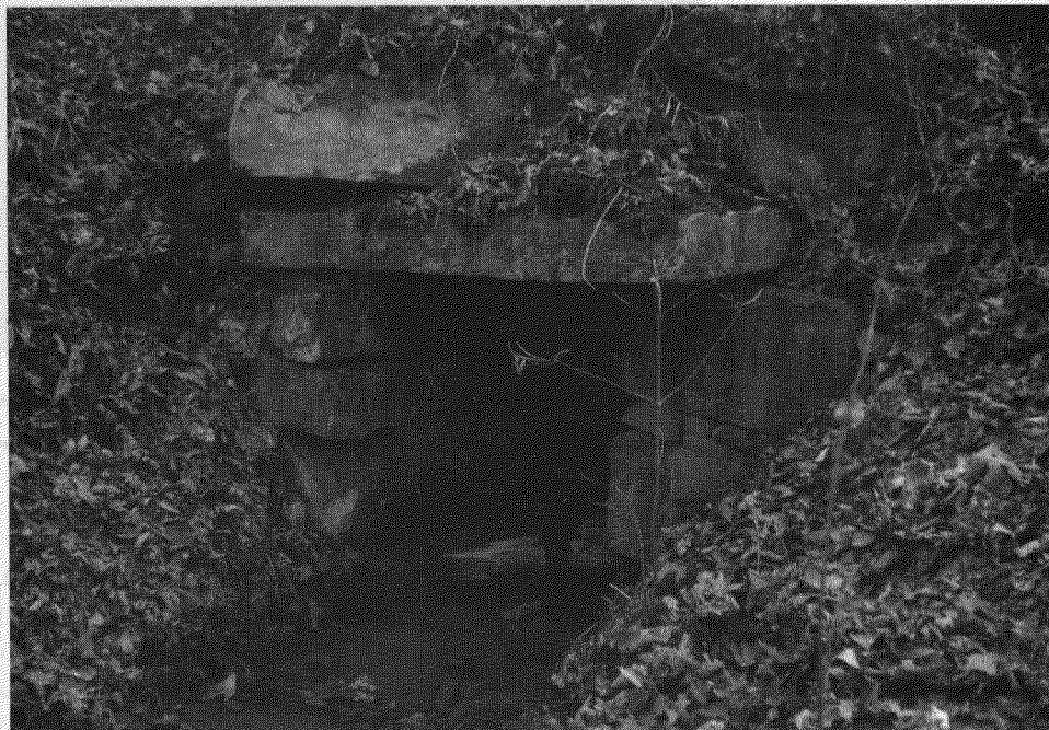
Figure 14.—CCC constructed rock slab box culvert.
