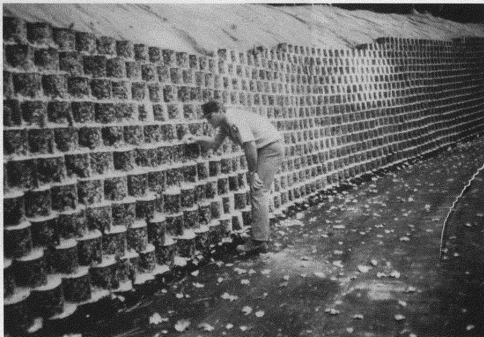
Figure 9.—Completed gravity wall. Note the undulating "top of cut" line.
