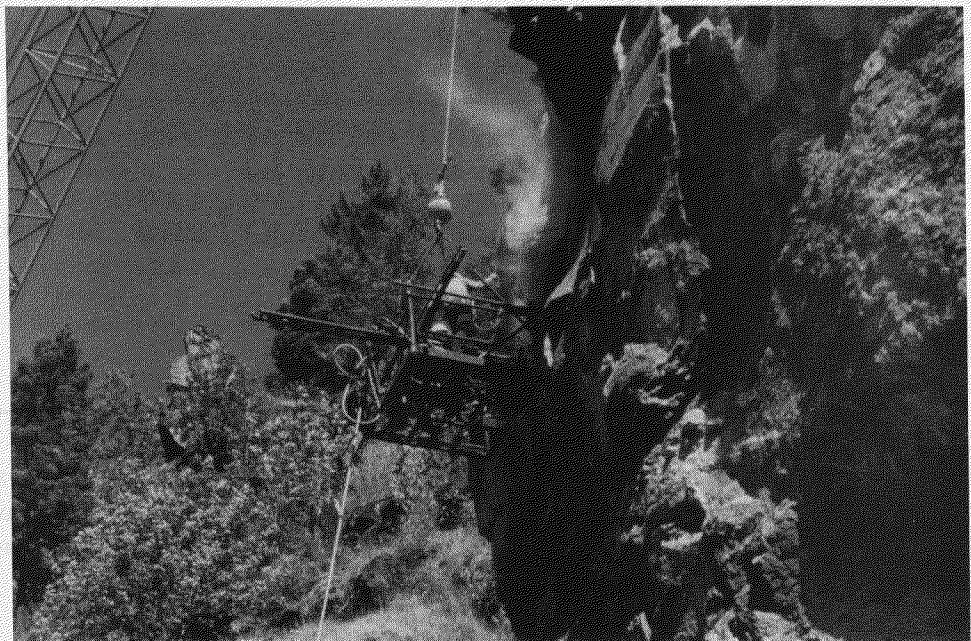
Figure 9.—Lift basket and drill used to install rock bolts.
