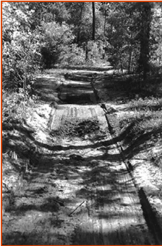
Figure 1—Evaluating equipment that effectively cuts the mounds and fills the depressions on washboard trails is what this report is about. This trail has been partly graded to remove the whoop-de-doo.
