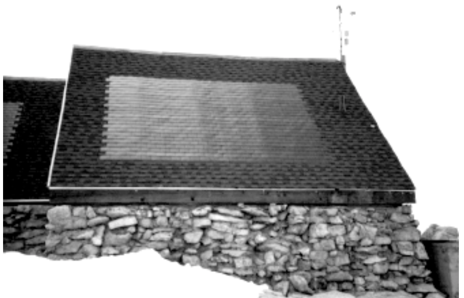
Figure 3—Photovoltaic shingles produce electricity on the roof of the Mt. Evans Observatory on the Roosevelt National Forest in Colorado. The system uses 48 shingles, each 7 feet long.
