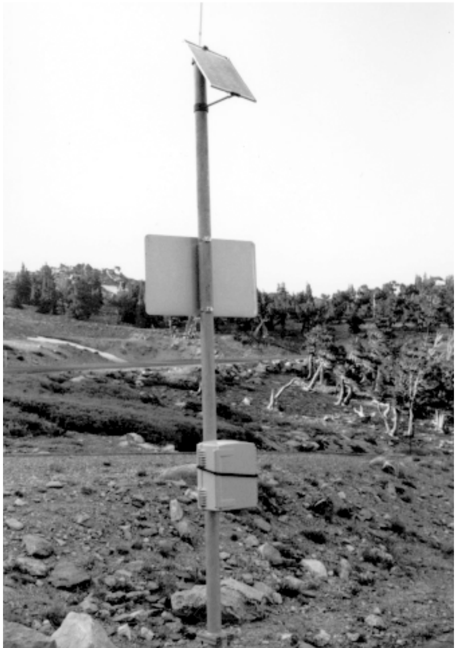
Figure 1—Photovoltaic systems are ideally suited when power is needed far from powerlines. This panel powers an emergency phone system along the road to Mt. Evans on the Roosevelt National Forest in Colorado. The Colorado Department of Transportation shared the costs.
