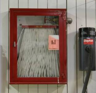
1910.157(d)(3) The employer may use uniformly spaced standpipe systems or hose stations connected to a sprinkler system installed for emergency use by employees instead of Class A portable fire extinguishers, provided that such systems meet the respective requirements of 1910.158 or 1910.159, that they provide total coverage of the area to be protected, and that employees are trained at least annually in their use.
