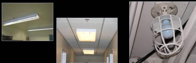
**1910.305(a)(2)(iii)(F)** Lamps for general illumination shall be protected from accidental contact or breakage. Protection shall be provided by elevation of at least 7 feet from normal working surface or by a suitable fixture or lampholder with a guard.
