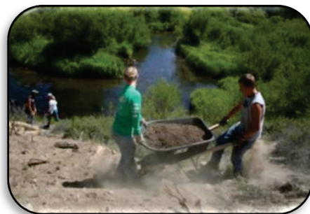
Figure 2. Crescent District employees mulching an eroding slope.
