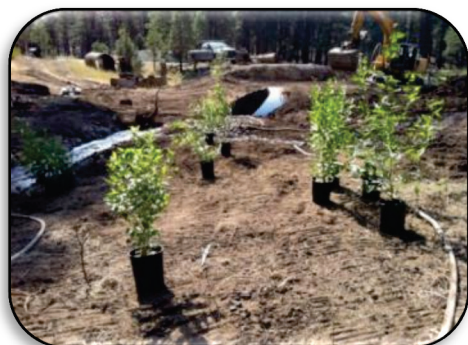
Figure 3. Black cottonwoods waiting to be planted at Sugar Creek Culvert Replacement Project, Paulina District, Ochoco NF.
