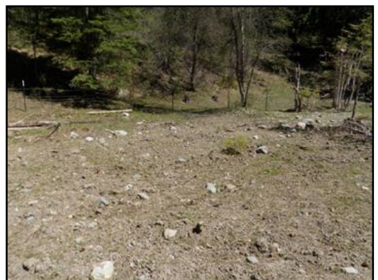
Figure 2. Restoration efforts near the Pierre Creek culvert replacement site, May 2013.
