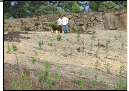
Foster Creek disposal area, North Umpqua Highway Project.
