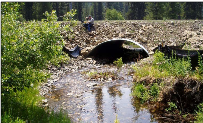
Figure 2. Restoration efforts at a culvert replacement project.
