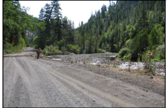
Figure 2. Hydrologist Stacia Peterson raking in native seed at road 32 reconstruction site on Walla Walla District. Photo by Joan Frazee.
