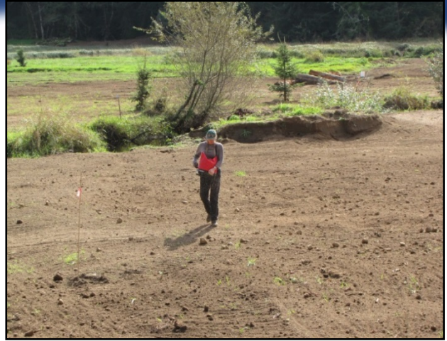
Figure1. Riparian Restoration. Seeding native species on a recently graded portion of the 80 acre Five Mile-Bell riparian restoration project.
