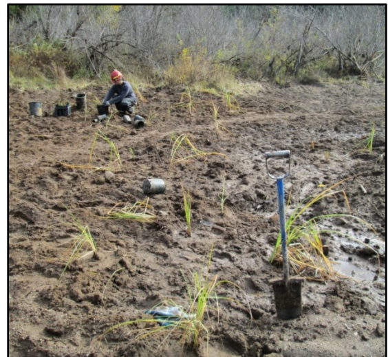
Figure 2. Sedges being planted in the wetland area of Stump Lake in the early fall of 2014.
