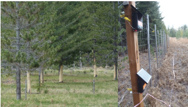
Coyote seed orchard bear damaged trees and electrified fence installed to prevent future damage Photos: A. Bower & R. Watson
