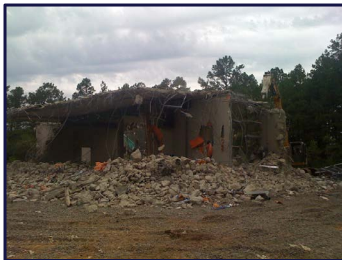
Figure 1. American Tower being torn down and removed.
